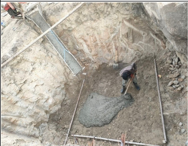
Lean concrete the TA-160 leg A,B.
