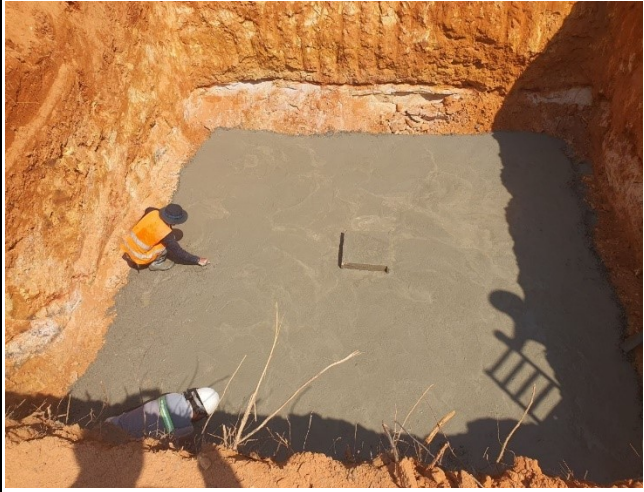
Lean concrete of leg A
