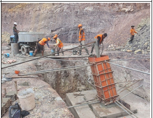
Chimney concrete and leveling of leg B.
