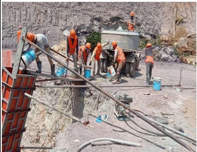
Chimney concrete and compaction of leg C.
