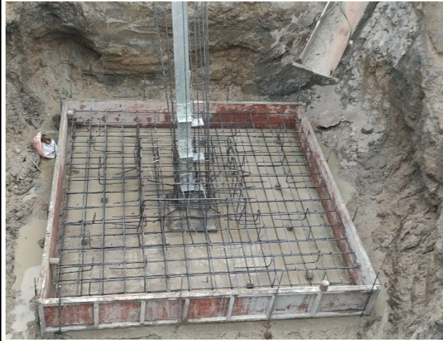
Base rebar arrangement and formwork installation of leg D.
