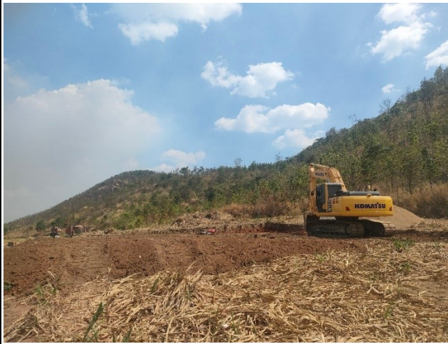
Soil excavation of leg A,C,D.
