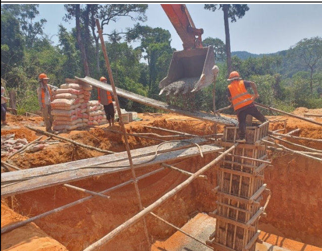
Chimney concrete and leveling of leg C.
