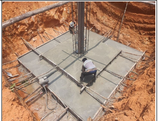
Base concrete and leveling of leg C.
