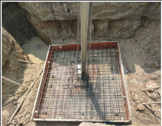
Base rebar arrangement and formwork installation of leg B.
