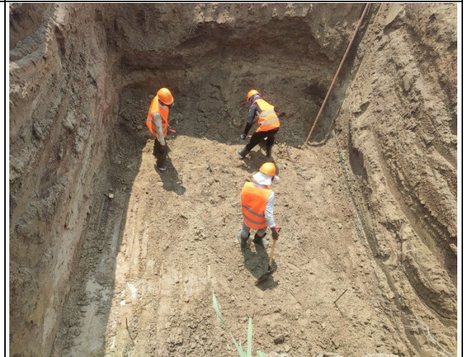
Soil leveling of leg C&D
