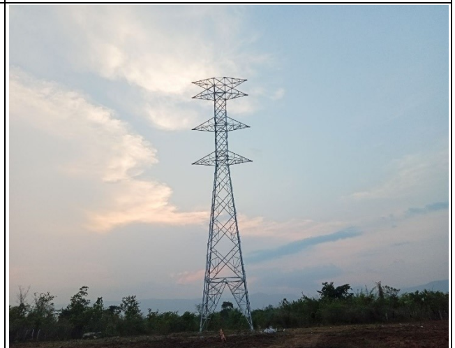
Tower erection of TB-15
