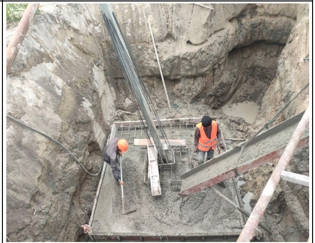
Base concrete and compaction of leg B.
