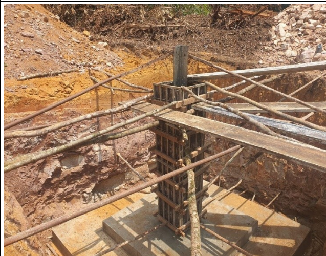
Chimney concrete and compaction of leg C
