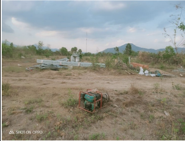
Tower erection of TB-14
