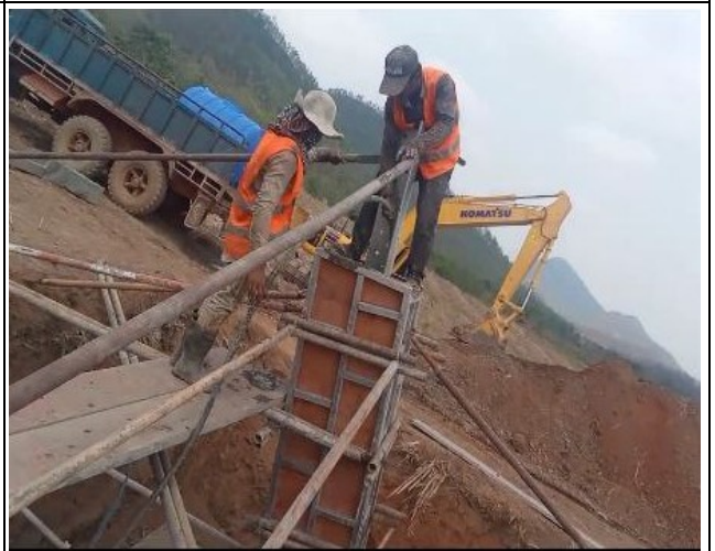
Chimney concrete and leveling of leg B,C.
