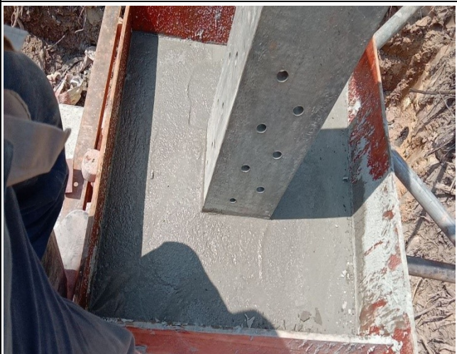
Chimney concrete and leveling of leg C.
