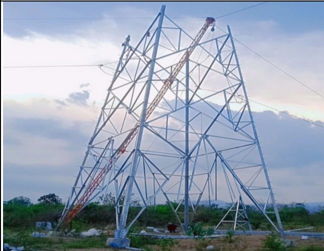
Tower erection of TB-14
