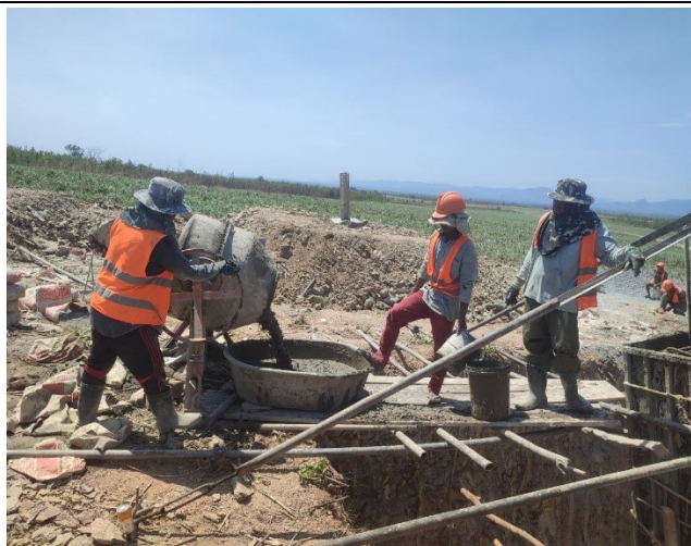
Chimney concreting of leg B.
