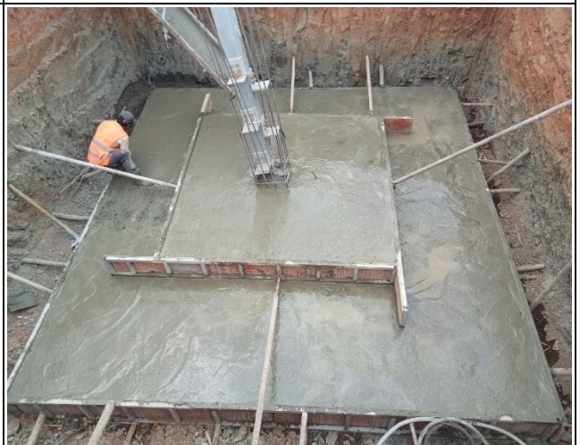
Base concrete and leveling of leg B.
