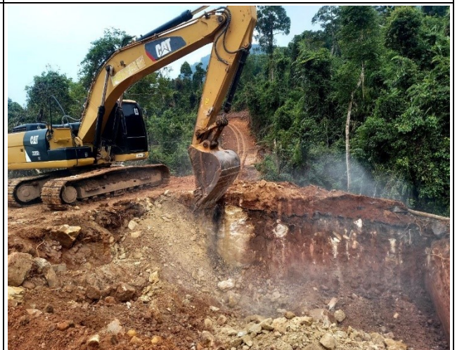
Soil excavation of leg A
