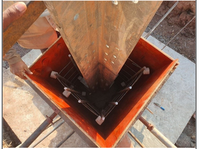
Chimney rebar arrangement & formwork installation of leg D.
