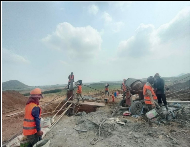
Chimney concrete and compaction of leg B,C.
