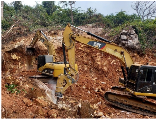
Soil cut of level location TB052
