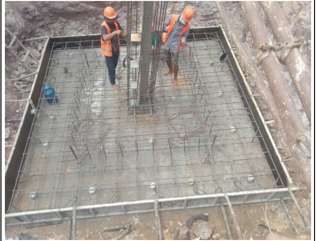
Rebar arrangement and formwork installation of leg B
