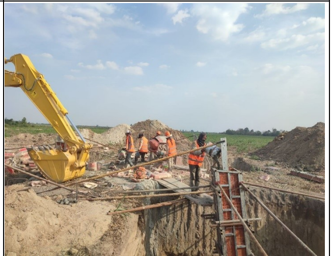
Chimney concrete of leg D.
