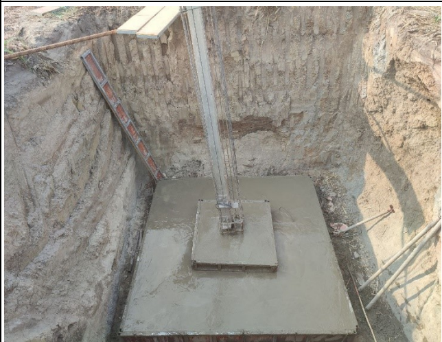
Base concrete and leveling of leg B.
