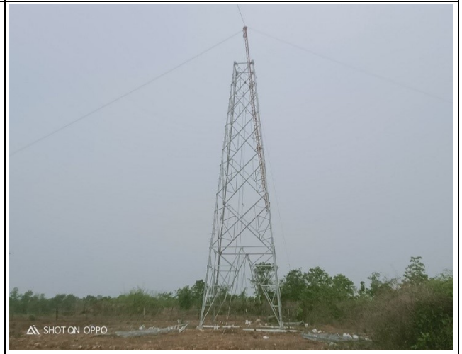
Tower erection of TB-15
