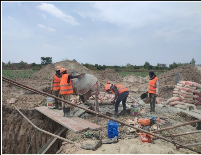
Chimney concrete mixing of leg B.
