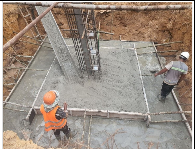
Concrete leveling of leg A
