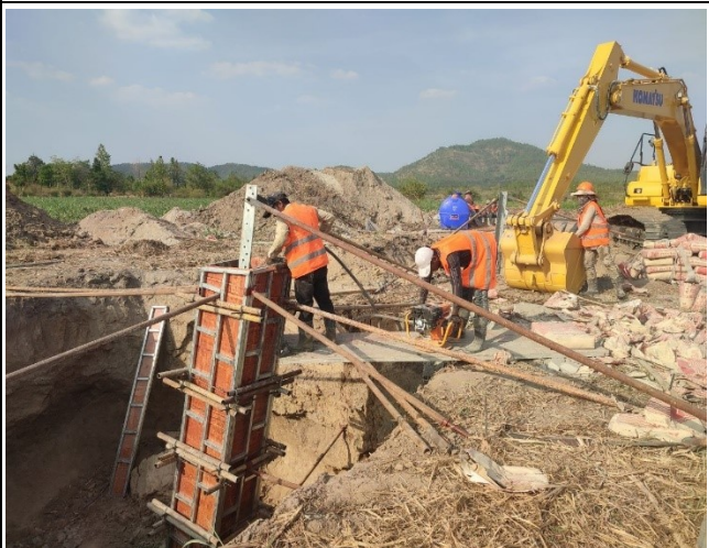
Chimney concrete and compaction of leg B.
