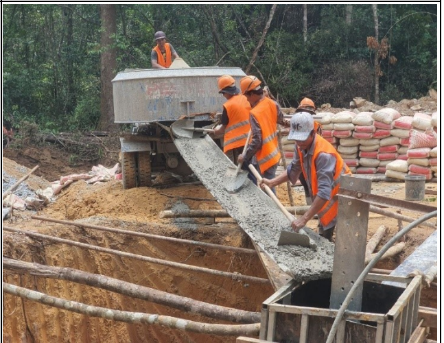
Chimney concrete and leveling of leg C
