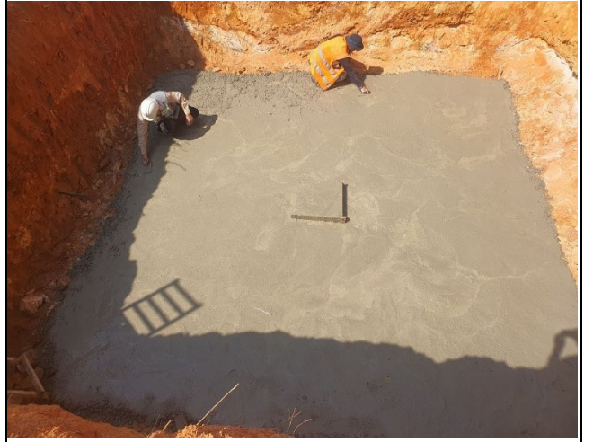
Lean concrete of leg B
