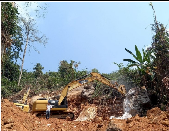
Soil cut of level location TB052
