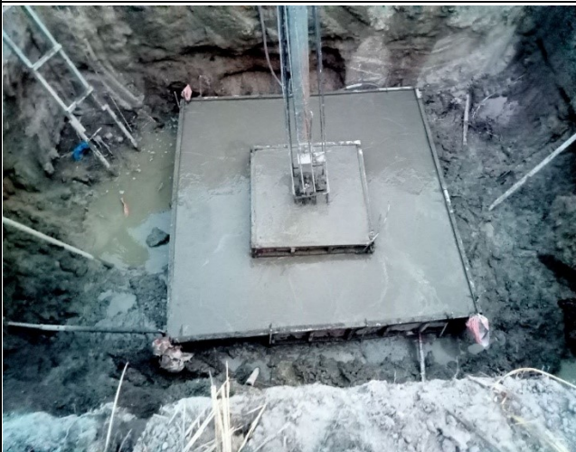
Base concrete and leveling of leg D.
