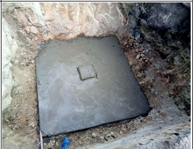
Lean concrete the TA-160 leg A,B.
