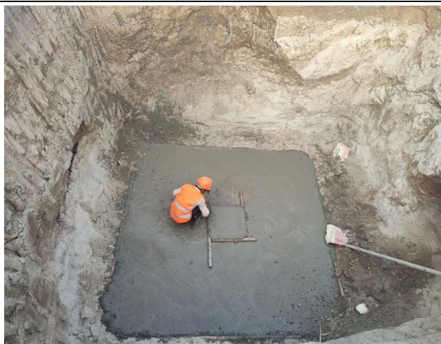
Lean concreting of leg A&B.
