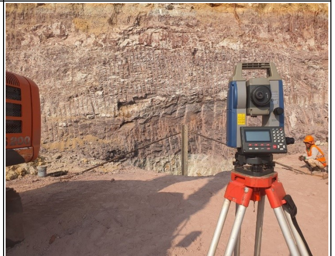
Stub setting of leg A.
