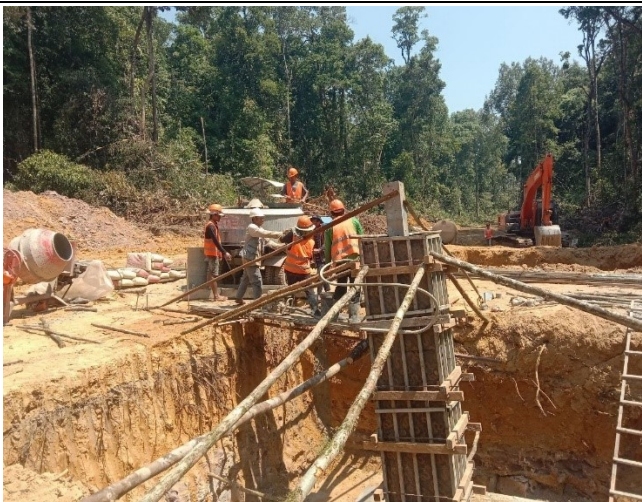
Chimney concrete and compaction of leg A
