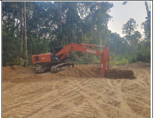
Soil excavation of leg B.
