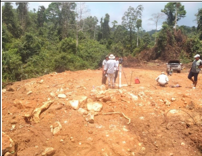
Setting out point of leg A,B,C,D
