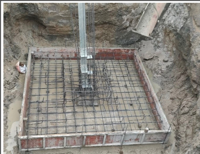
Base rebar arrangement and formwork installation of leg C.
