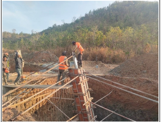
Chimney concrete and compaction of leg A.
