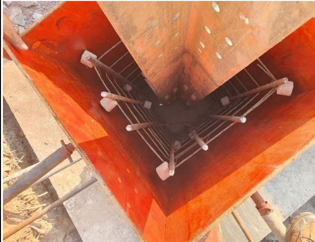
Chimney rebar arrangement & formwork installation of leg C.
