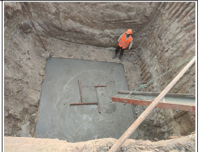
Lean concreting of leg C&D.
