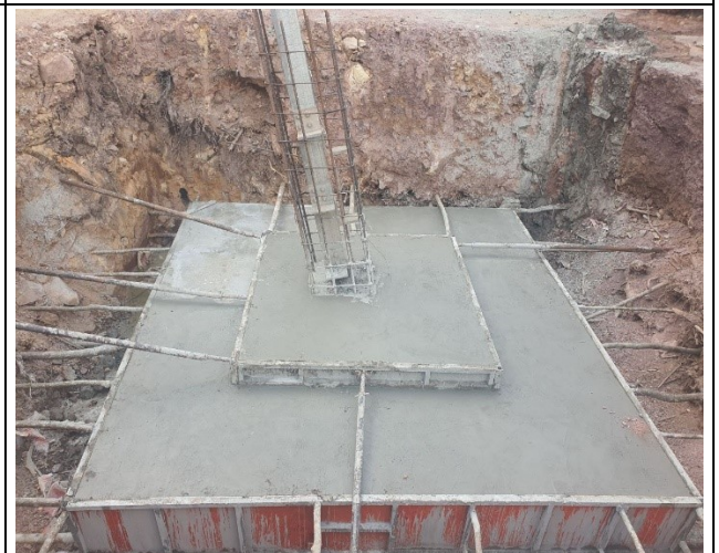
Base concrete and leveling of leg D.
