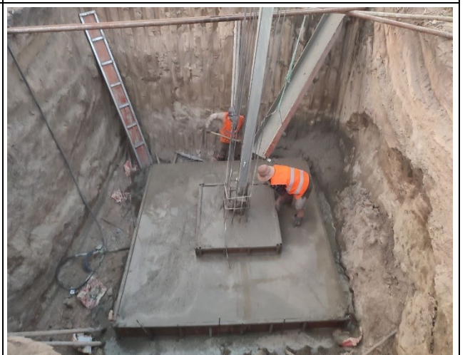
Base concrete and leveling of leg C.
