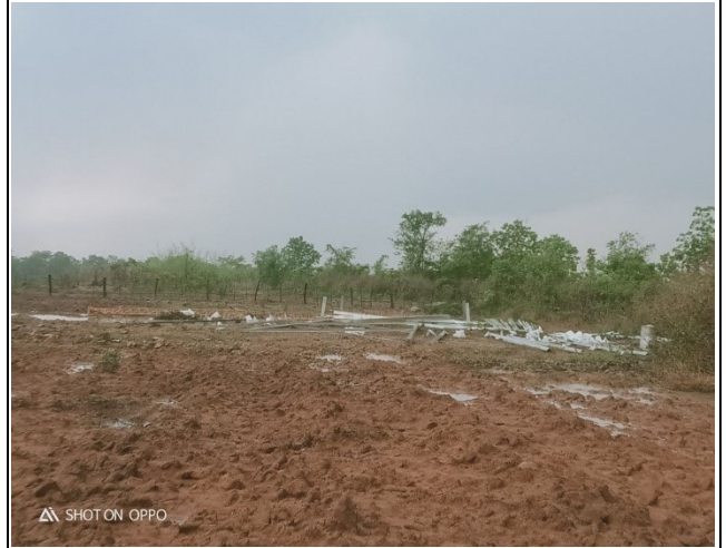
Tower erection of TB-15
