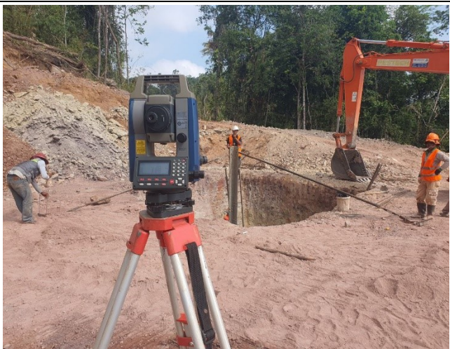
Stub setting of leg B
