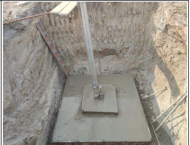
Base concrete and leveling of leg D.
