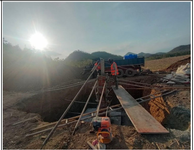
Chimney concrete of leg A.
