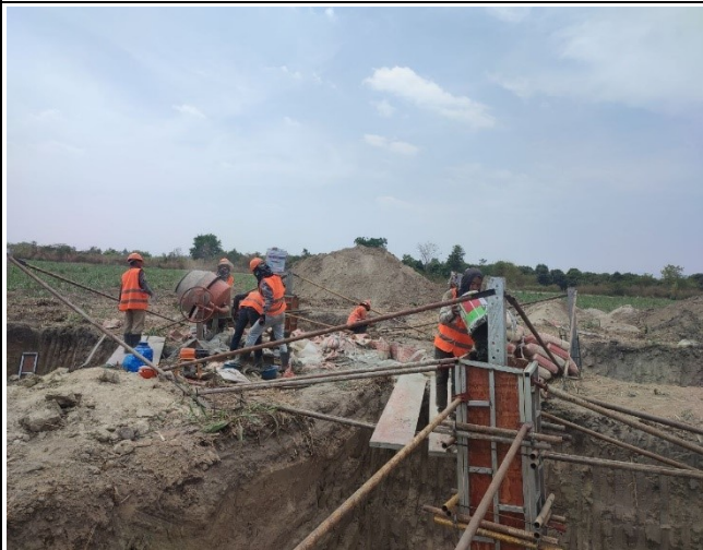
Chimney concrete of leg B.
