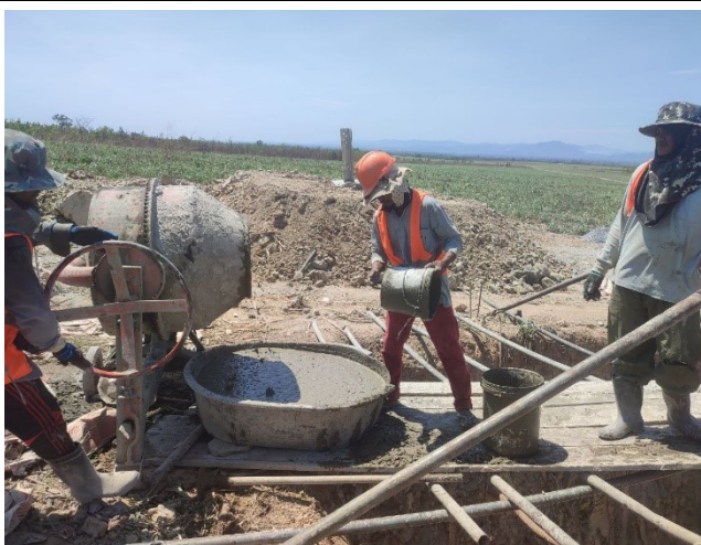
Chimney concreting of leg B.
