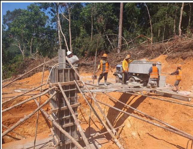
Chimney concrete and leveling of leg B.
