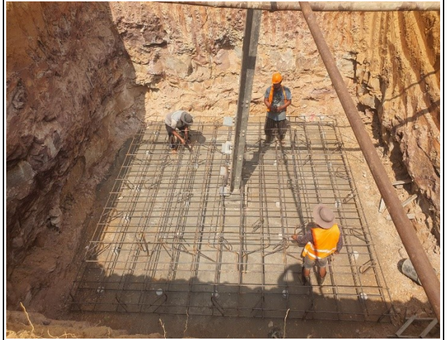
Base rebar arrangement of leg D
