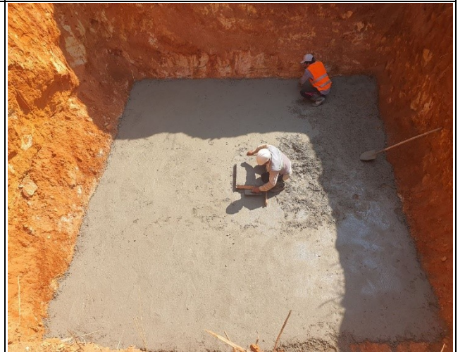
Lean concrete of leg D
