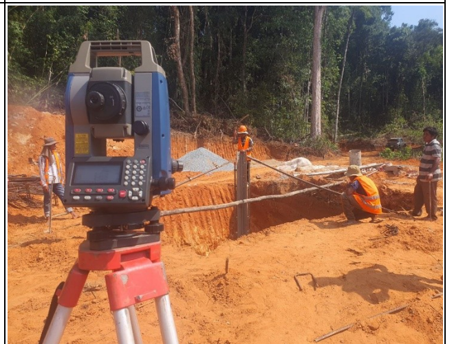
Stub setting of leg C,D
