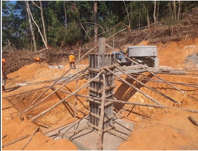
Chimney rebar arrangement and formwork installation of leg B.
