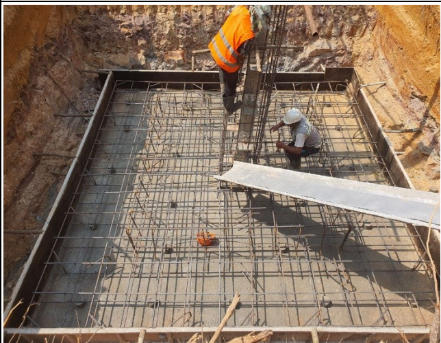
Rebar arrangement & formwork installation of leg A
