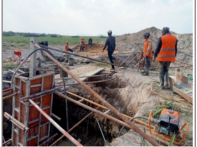
Chimney rebar arrangement and formwork installation of leg A,B.
