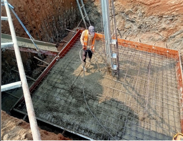
Base concrete and compaction of leg A.
