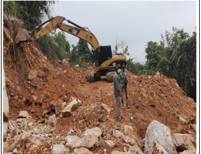
Soil cut of level location TB052
