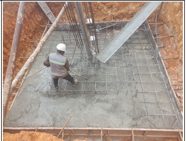
Base concrete and compaction of leg B.
