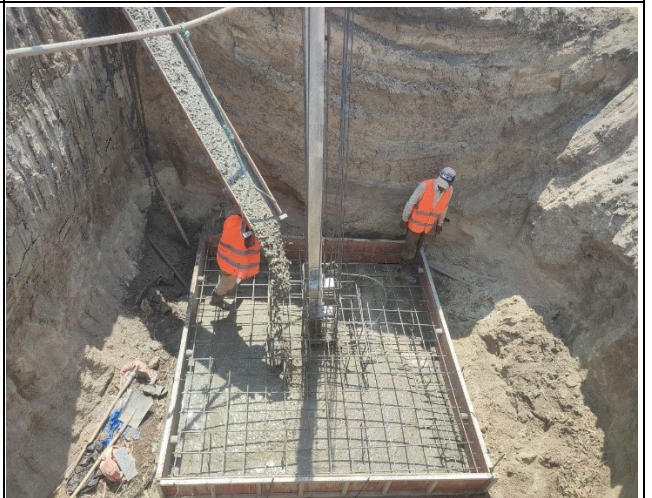
Base concrete and compaction of leg A.
