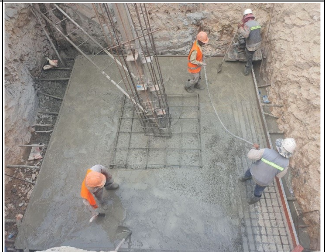
Base concrete and compaction of leg D.
