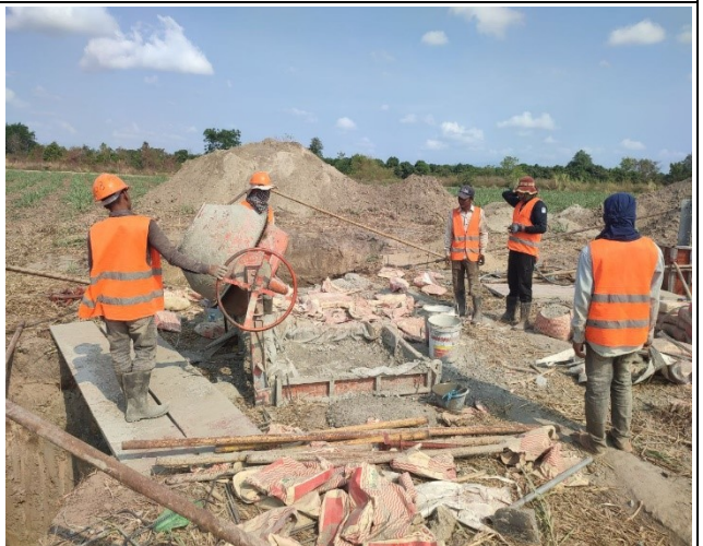
Chimney concrete mixing and casting of leg C.
