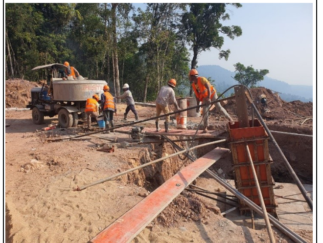
Chimney concrete and compaction of leg D.
