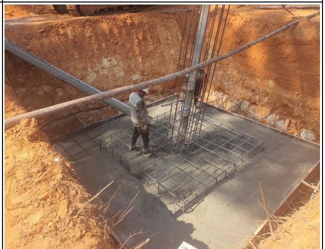
Base concrete and leveling of leg B.
