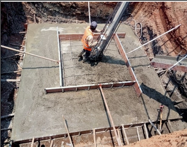
Base concrete of leg A.
