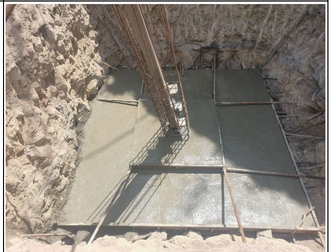
Base concrete and leveling of leg A.
