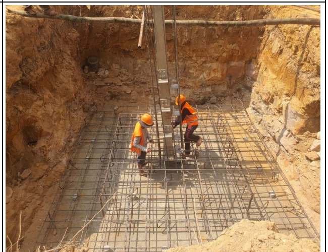
Base rebar arrangement of leg C
