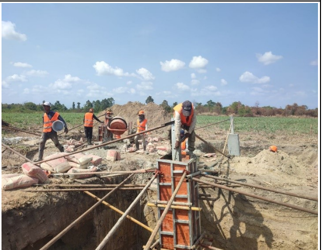
Chimney concrete and compaction of leg C.
