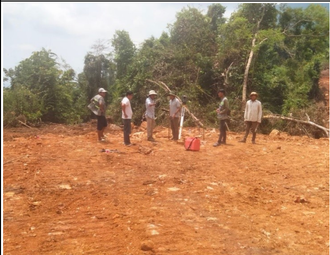
Setting out point of leg A,B,C,D
