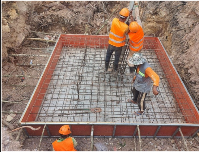
Base rebar arrangement&formwork installation of leg C.
