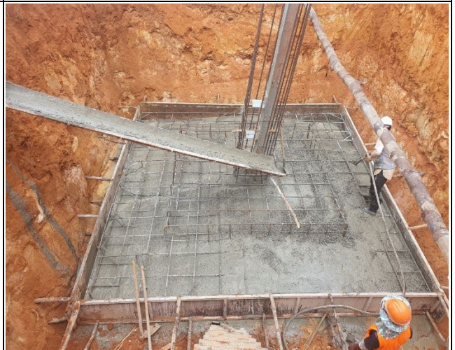
Base concrete and compaction of leg A.
