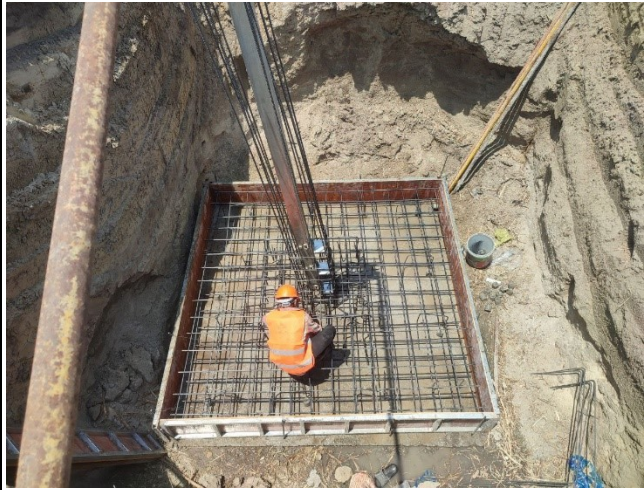
Base rebar arrangement & formwork installation of leg A.
