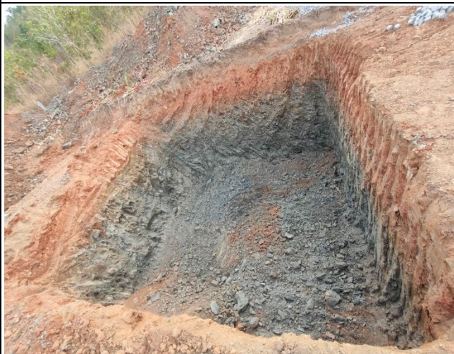
Soil excavation of leg A,C,D.
