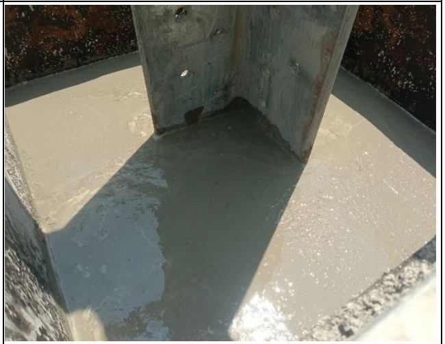
Concrete leveling of leg A
