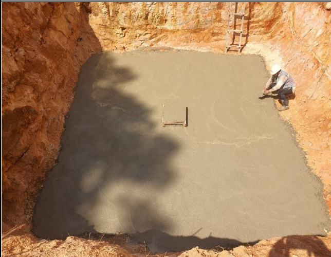
Lean concrete of leg C
