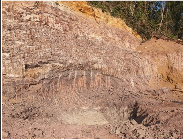
Soil excavation of leg A.
