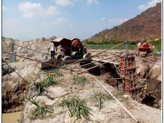
Chimney rebar arrangement and formwork installation of leg D.
