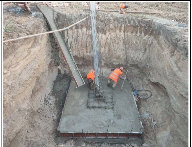
Base concrete and compaction of leg D.
