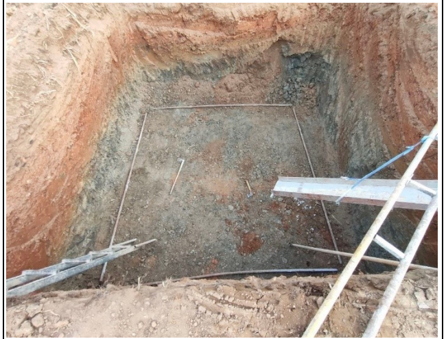
Lean concrete of leg A.
