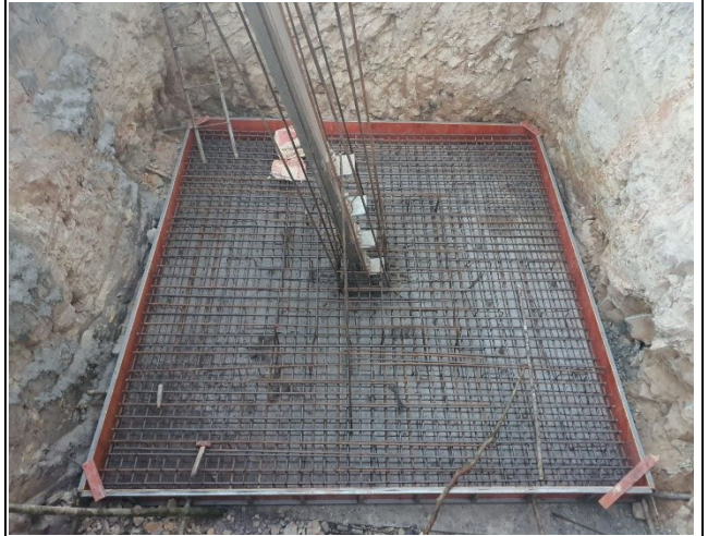
Base rebar arrangement&formwork installation of leg D.
