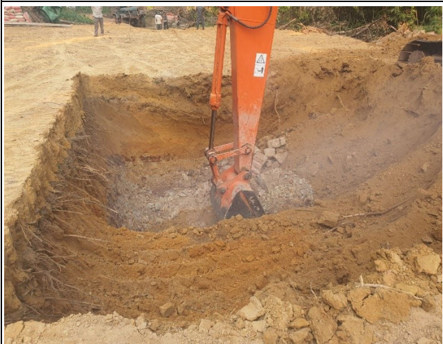
Soil excavation of leg A.
