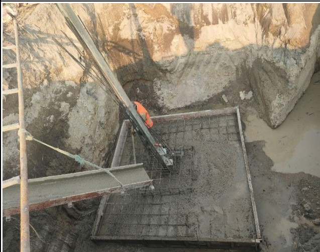
Base concrete and compaction of leg D.
