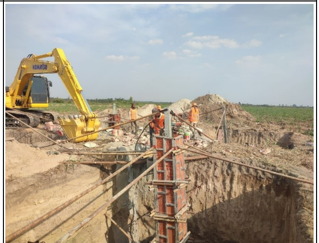
Chimney concrete and compaction of leg D.
