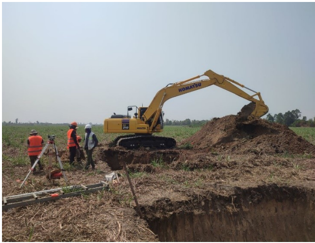
Soil excavation of leg A&B
