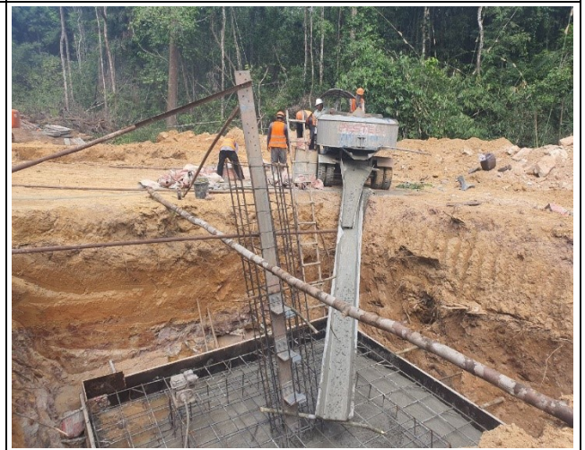
Casting concrete of leg A
