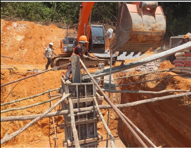
Chimney concrete and compaction of leg C.
