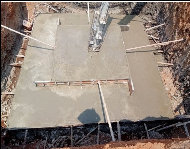
Base concrete and leveling of leg A.
