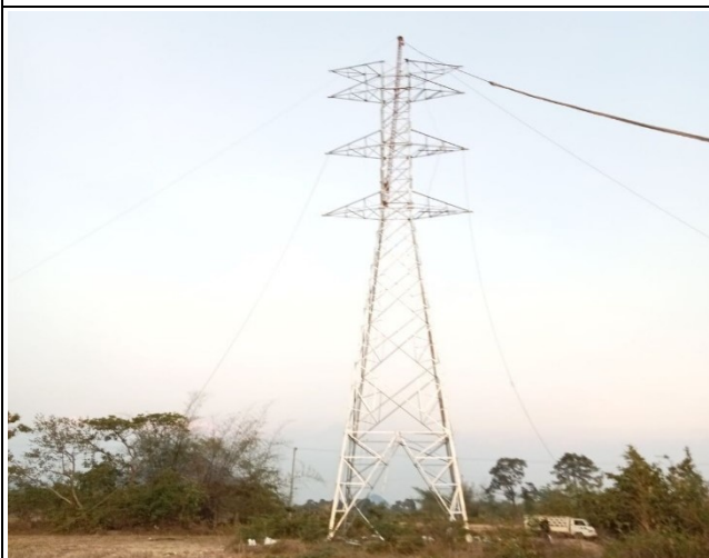
Tower erection of TB-13
