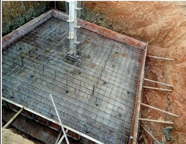
Stub setting & Base rebar arrangement and formwork installation of leg C.
