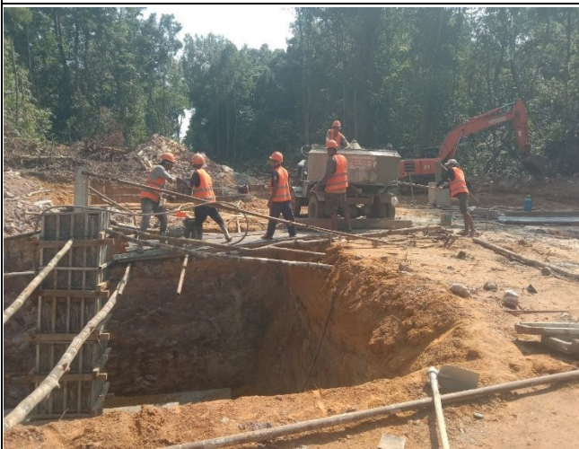
Chimney concrete and compaction of leg B
