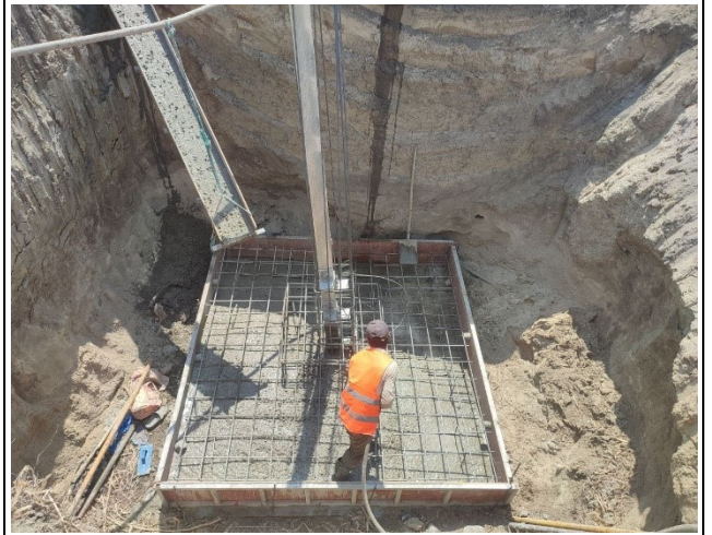
Base rebar arrangement & formwork installation of leg C.
