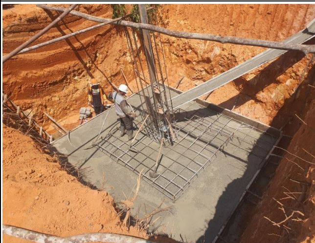
Base concrete and compaction of leg C.
