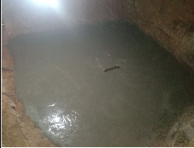
Lean concreting of leg A
