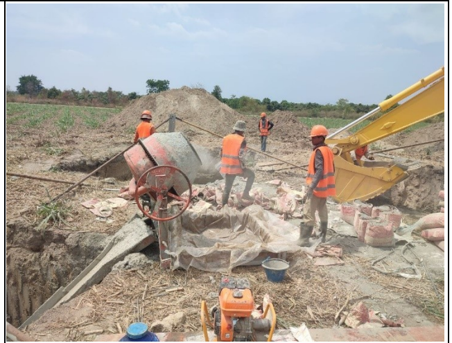
Chimney concrete mixing of leg D.
