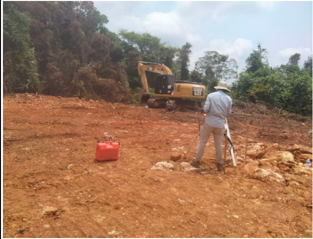
Setting out point of leg A,B,C,D
