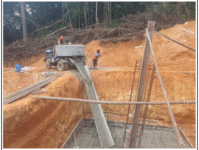
Base concrete of leg B.
