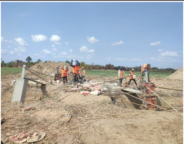
Chimney concrete mixing and casting of leg A.
