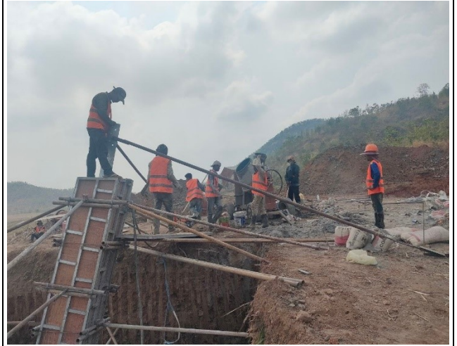
Chimney concrete and compaction of leg B,C.
