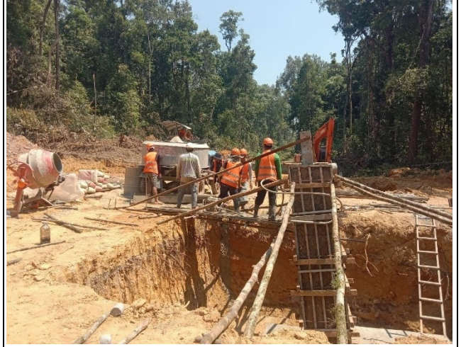
Concrete mixing of leg A
