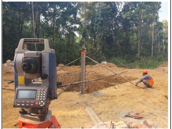
Stub setting of leg A
