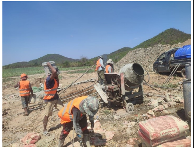
Concrete mixing for casting of leg B
