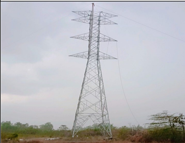
Tower erection of TB-14
