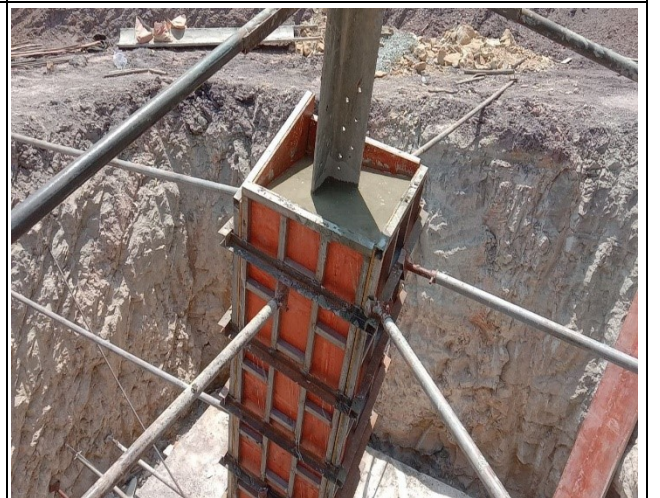
Chimney concrete and leveling of leg D.
