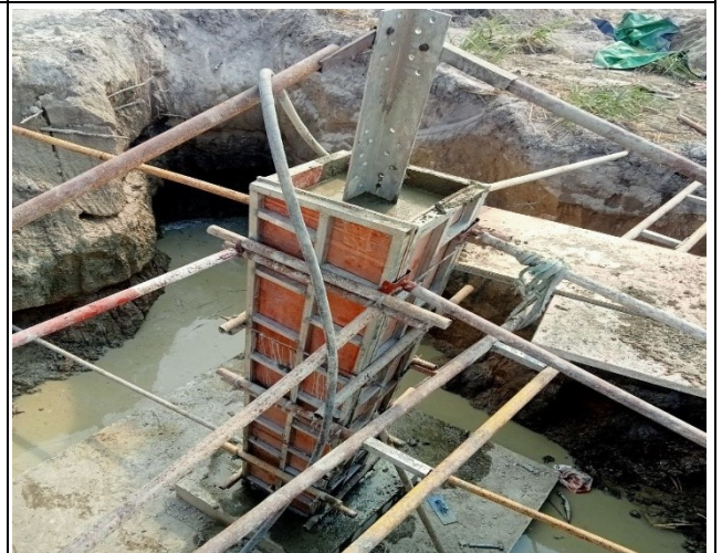
Chimney concrete and leveling of leg A,B.
