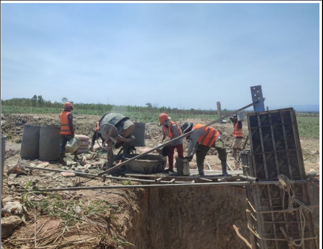
Chimney concreting of leg B.
