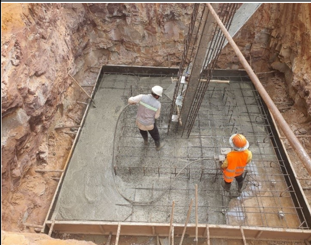
Base concrete and compaction of leg B
