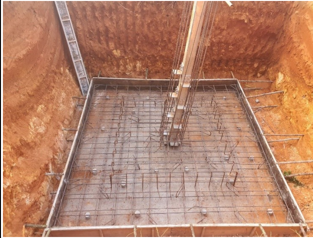
Base rebar arrangement and formwork installation of leg A.
