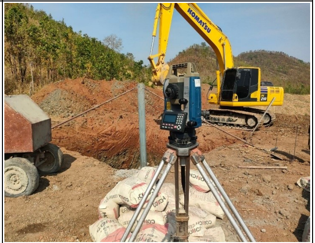
Stub setting of leg A.
