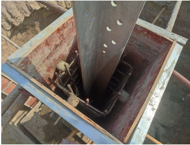
Chimney rebar arrangement and formwork installation of leg A.
