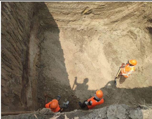
Soil leveling of leg A&B
