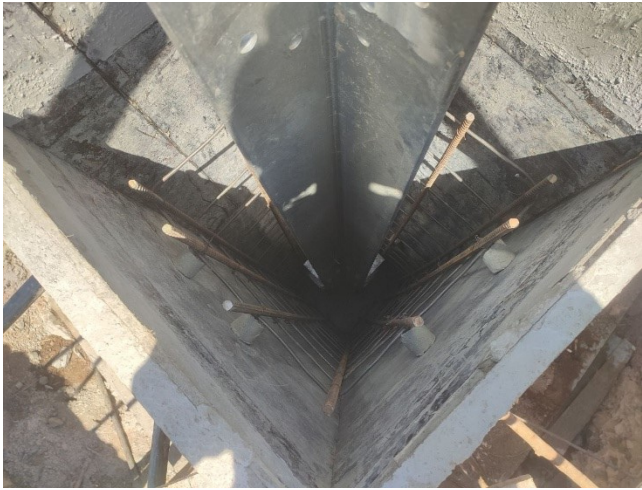
Arrangement rebar & installation formwork Of leg B.
