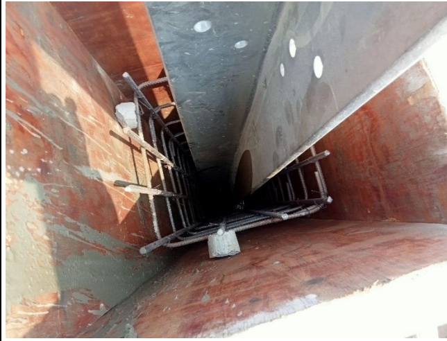
Chimney rebar arrangement and formwork installation of leg B,C.
