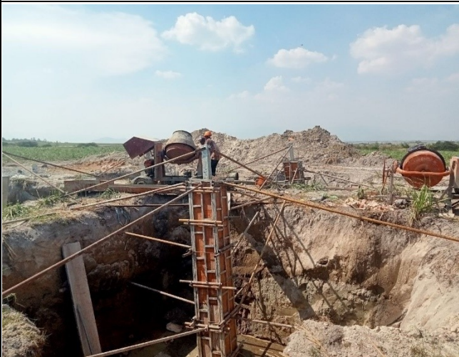
Chimney concrete and compaction of leg C.
