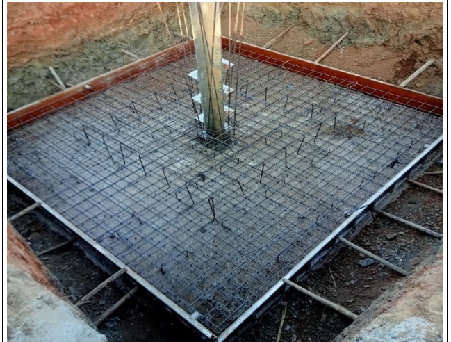
Base rebar arrangement and formwork installation of leg B.
