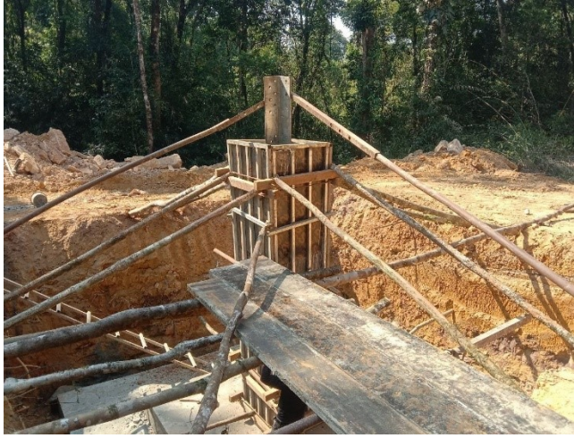
Chimney rebar arrangement & formwork installation of leg A
