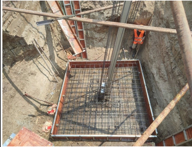
Base rebar arrangement & formwork installation of leg B.
