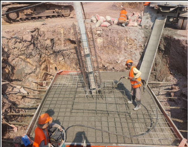
Base concrete and compaction of leg C.
