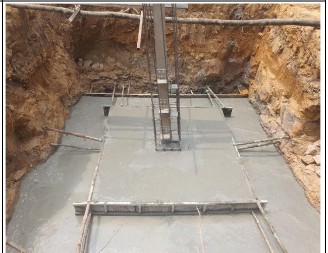
Concrete leveling of leg D
