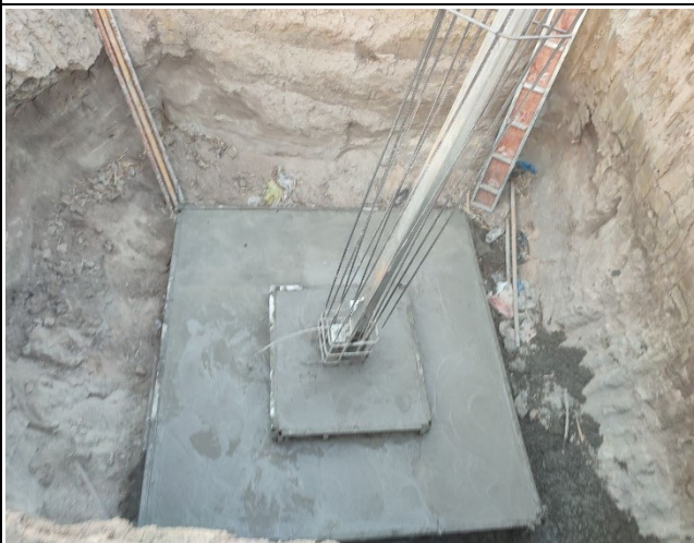
Base concrete and leveling of leg A.
