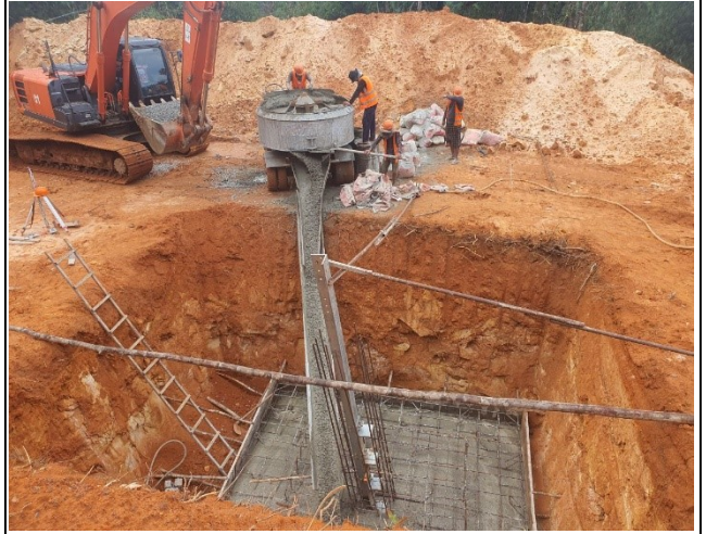
Base concrete of leg A.
