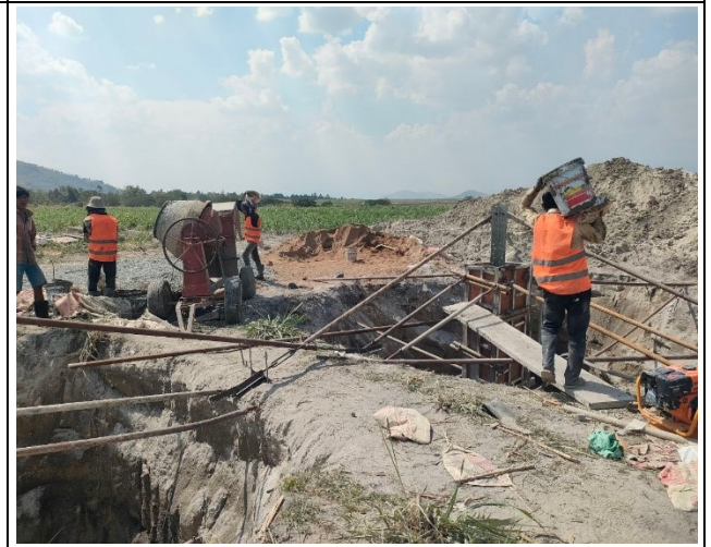
Chimney concrete and compaction of leg A,B.
