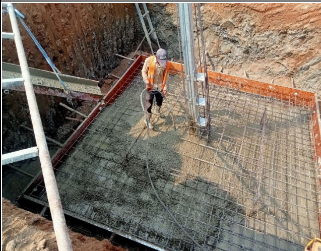
Base concrete and compaction of leg C.
