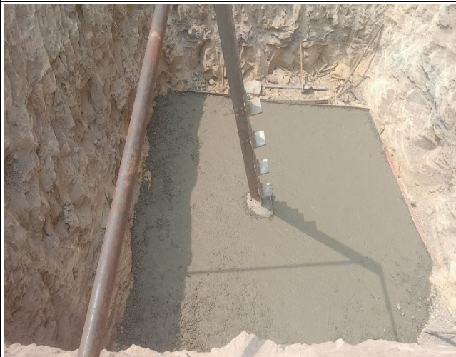
Lean concret of leg A.
