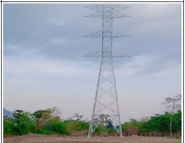
Tower erection of TB-12
