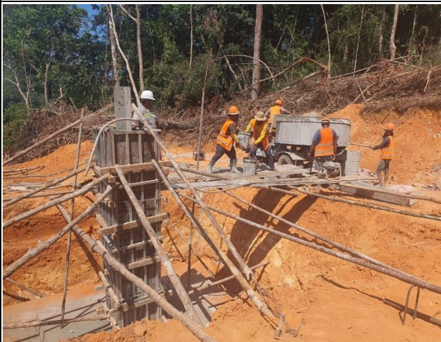
Chimney concrete and compaction of leg B.
