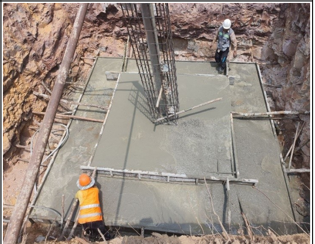
Concrete leveling of leg B
