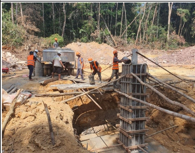
Chimney concret and compaction of leg D
