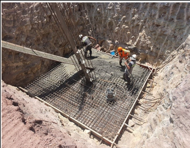
Base concrete of leg A.
