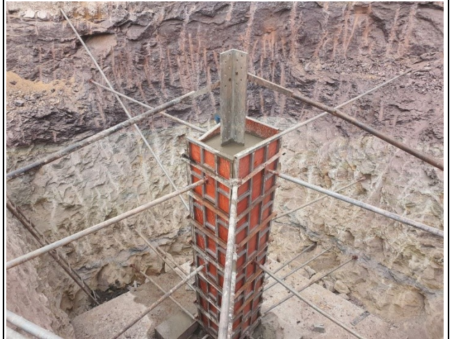
Concrete leveling of leg A.
