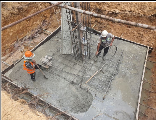
Concrete compaction of leg A
