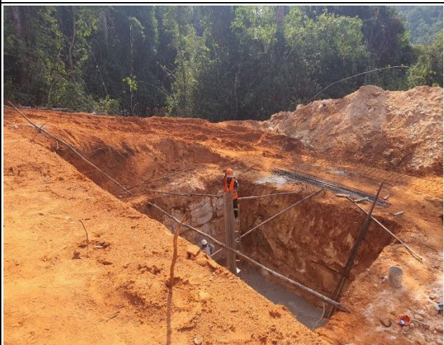
Stub setting of leg A,B
