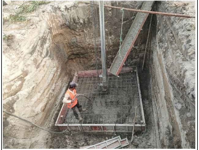
Base concrete and compaction of leg A.
