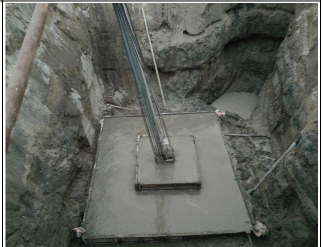
Base concrete and compaction of leg C.
