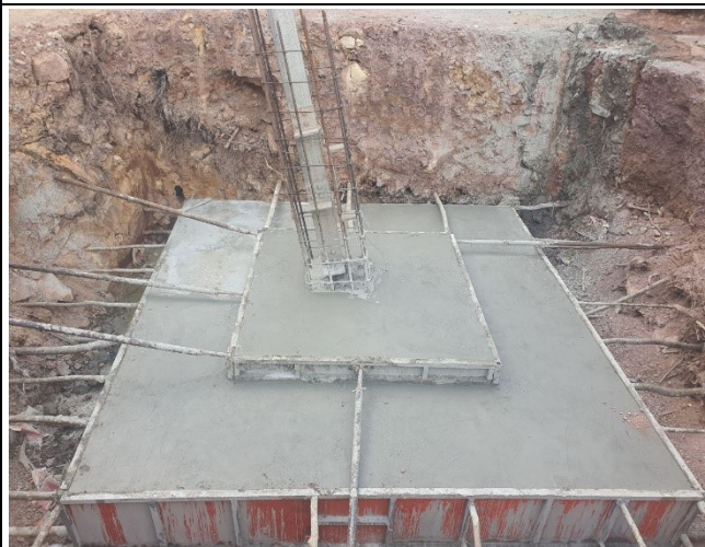
Base concrete and leveling of leg C.
