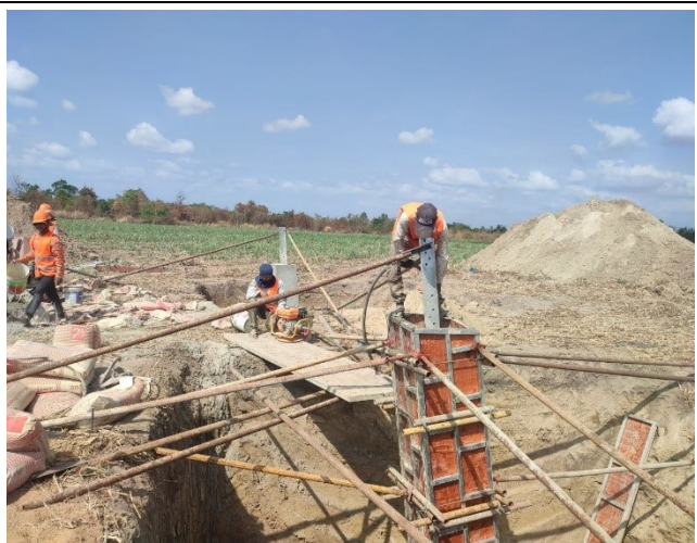
Chimney concrete and compaction of leg A.
