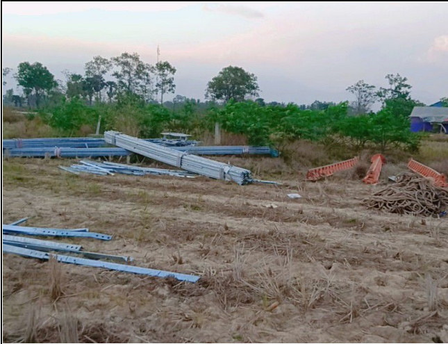
Tower erection of TB-13
