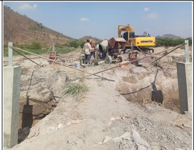
Chimney concrete and compaction of leg D.
