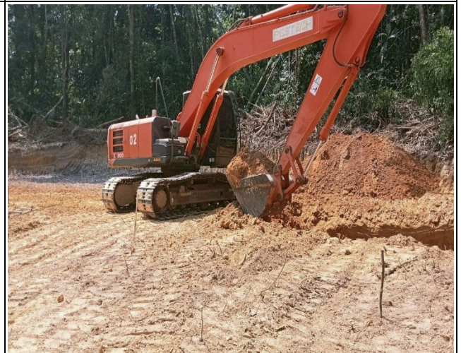
Soil excavation of leg D.
