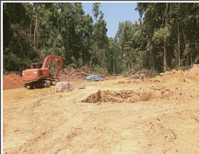
Soil excavation of leg C.
