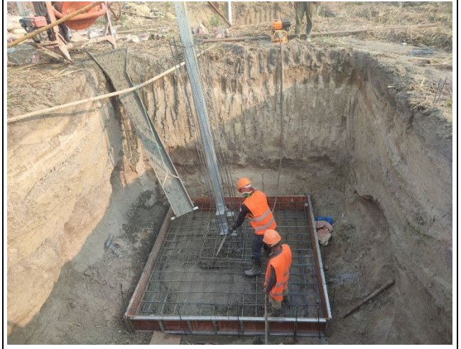
Base rebar arrangement & formwork installation of leg D.
