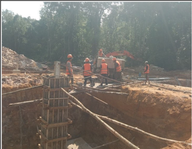
Chimney concrete mixing of leg B
