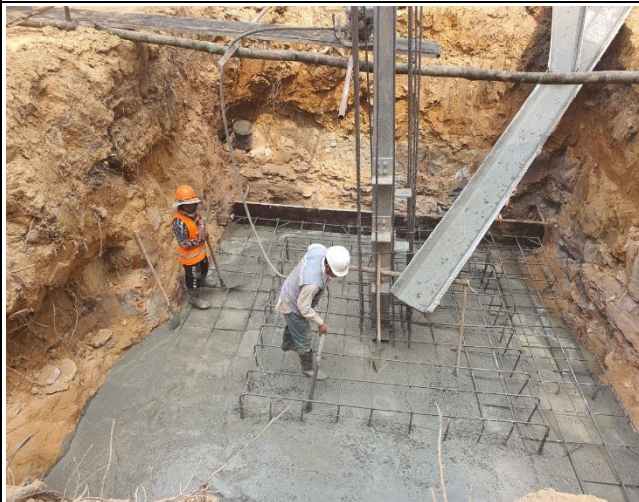
Base concret and compaction of leg D
