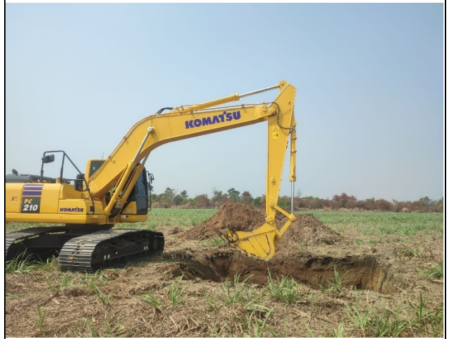
Soil excavation of leg C&D
