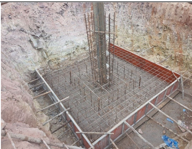
Formwork installation of leg B
