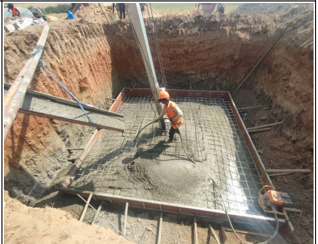
Base concrete and compaction of leg B.
