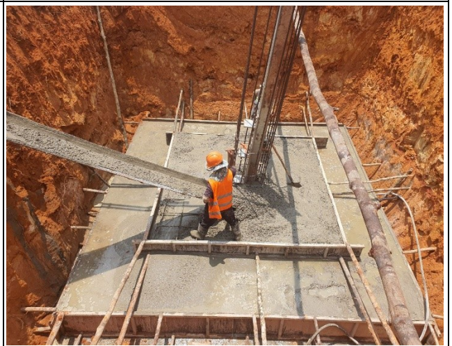
Base concrete and leveling of leg A.
