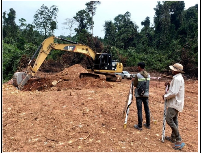
Soil excavation of leg A
