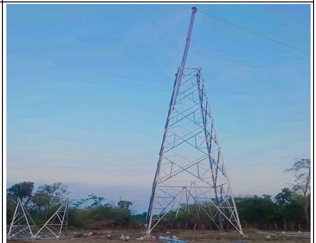
Tower erection of TB-12
