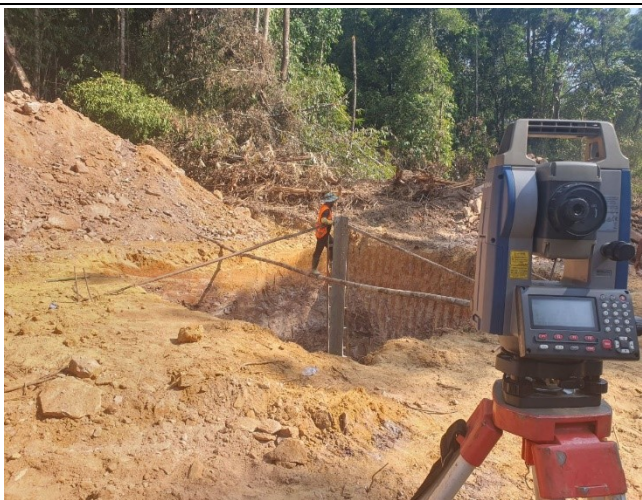
Stub setting of leg C
