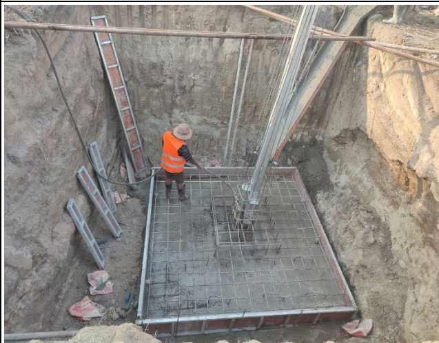
Base concrete and compaction of leg A.
