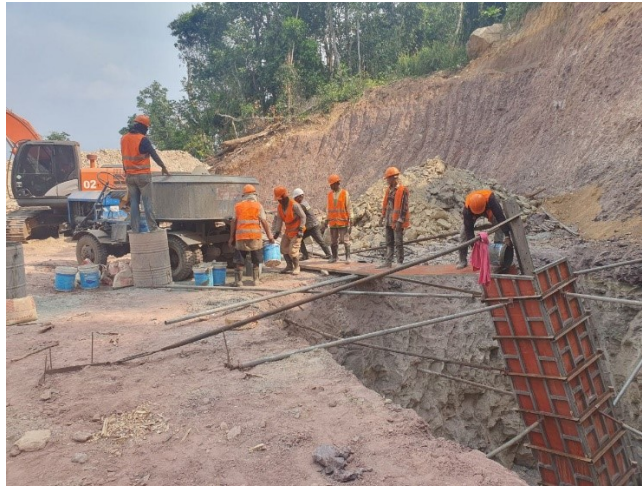
Chimney concrete and compaction of leg A.
