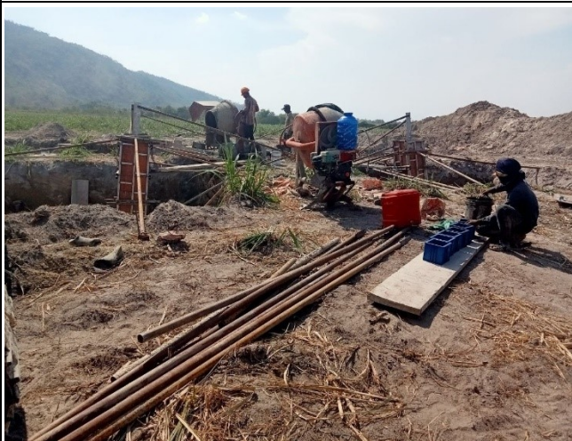
Chimney concrete and leveling of leg C
