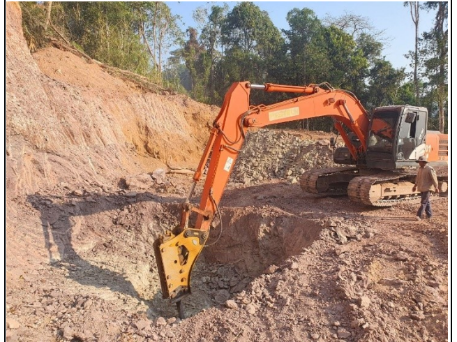
Rock breaking of leg A.
