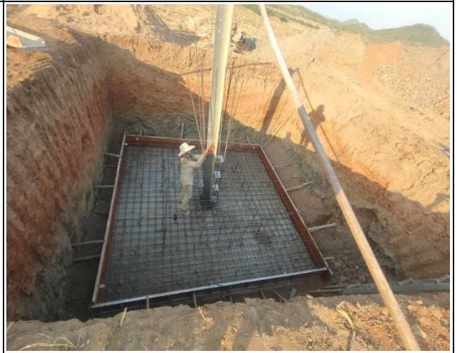
Stub setting and rebar arrangement of leg B.
