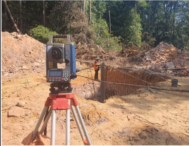
Stub setting of leg D
