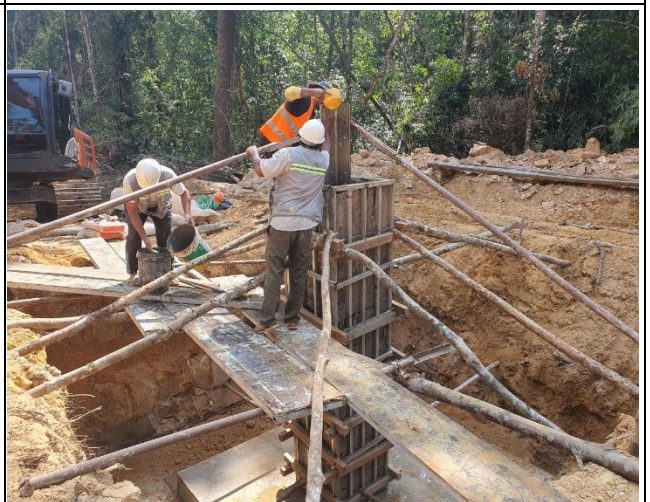
Chimney concrete and leveling of leg D
