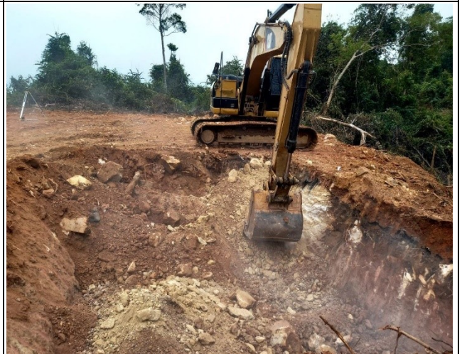
Soil excavation of leg A
