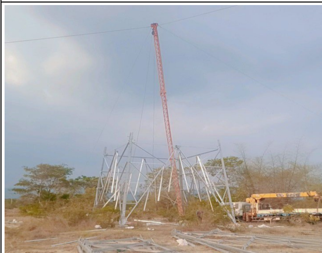
Tower erection of TB-13
