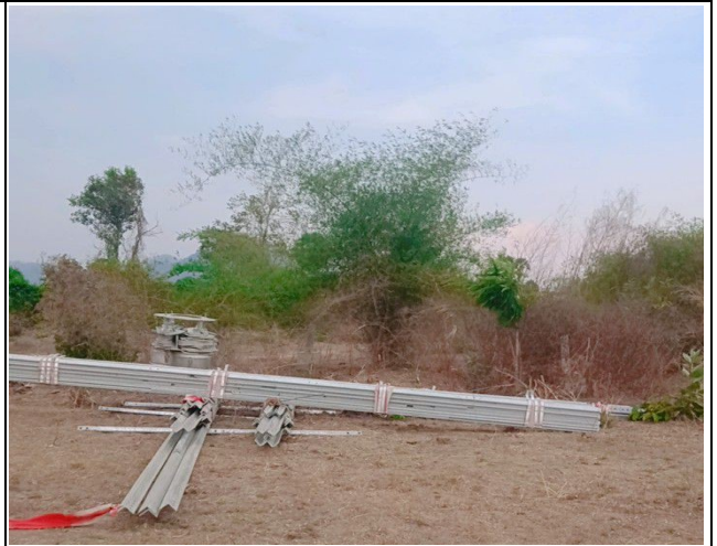
Tower erection of TB-12
