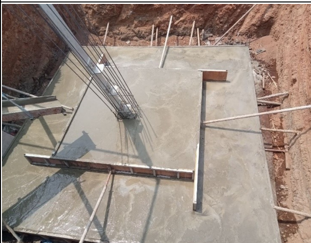
Base concrete and leveling of leg C.
