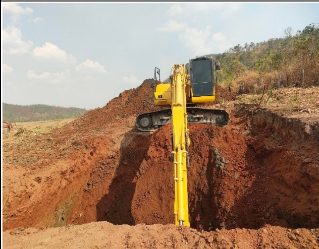
Soil excavation of leg A,C,D.
