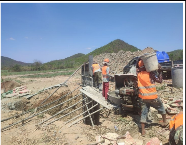
Chimney concreting of leg B.
