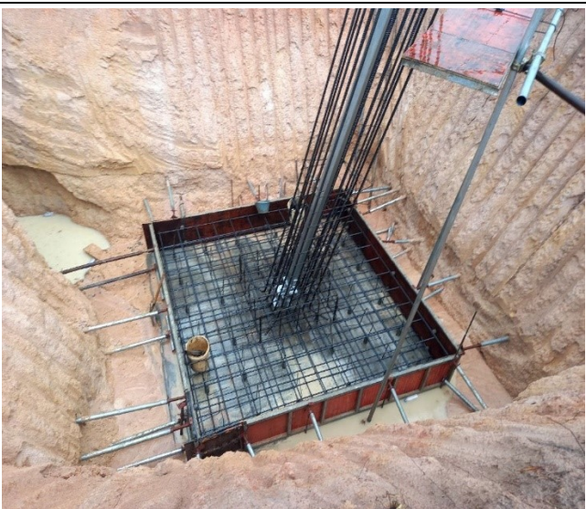
Base rebar & formwork installation leg A
