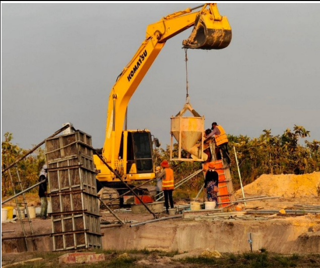
Chimney concrete leg D
