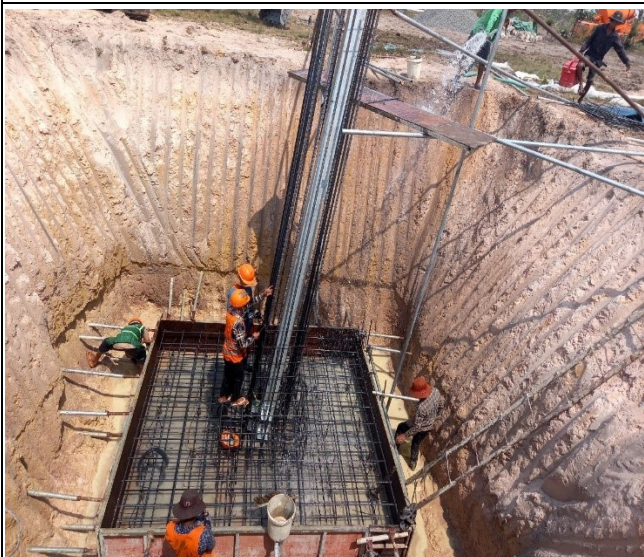
Base rebar & formwork installation leg B
