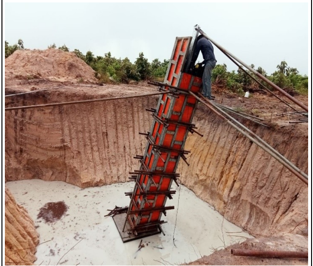
Stub setting leg C
