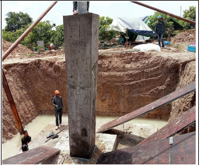
Remove form box leg C
