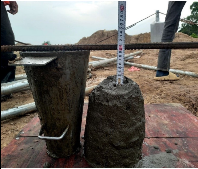
Slump testing leg A
