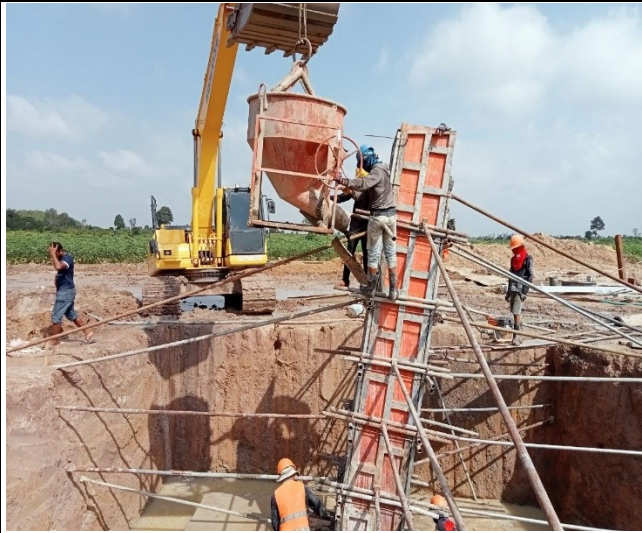
Chimney concrete leg D
