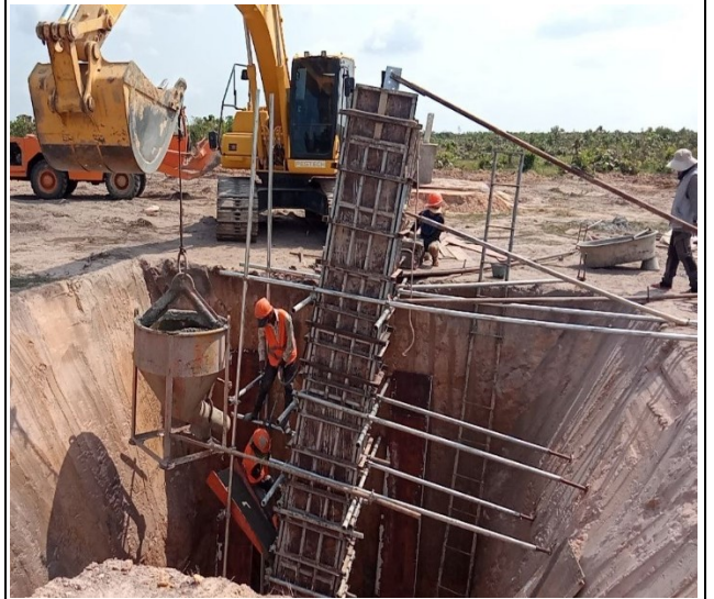
Chimney concrete leg A
