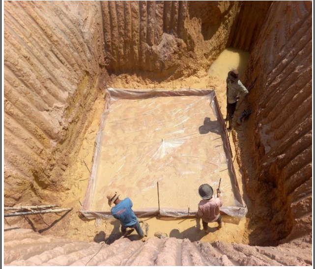
Lean concrete leg A
