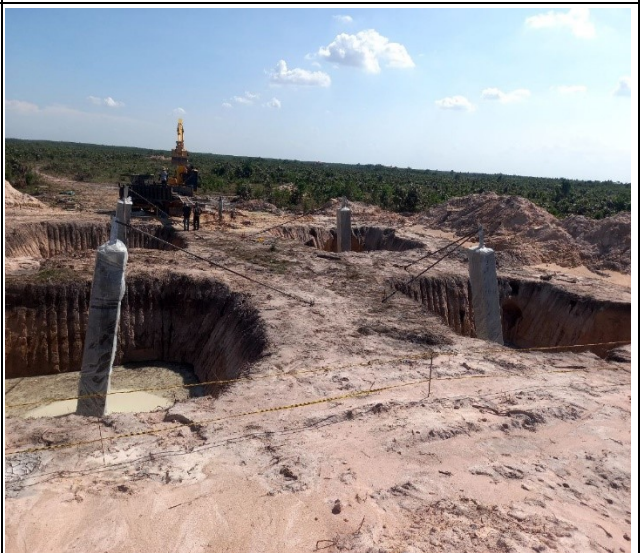
Remove chimney form box leg A
