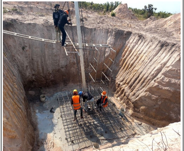
Base rebar installation leg C
