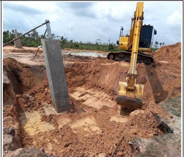
Backfill leg A
