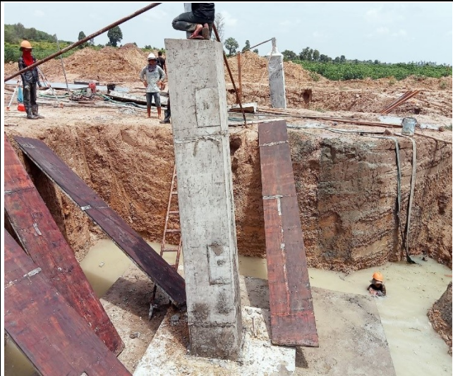
Remove form box leg C
