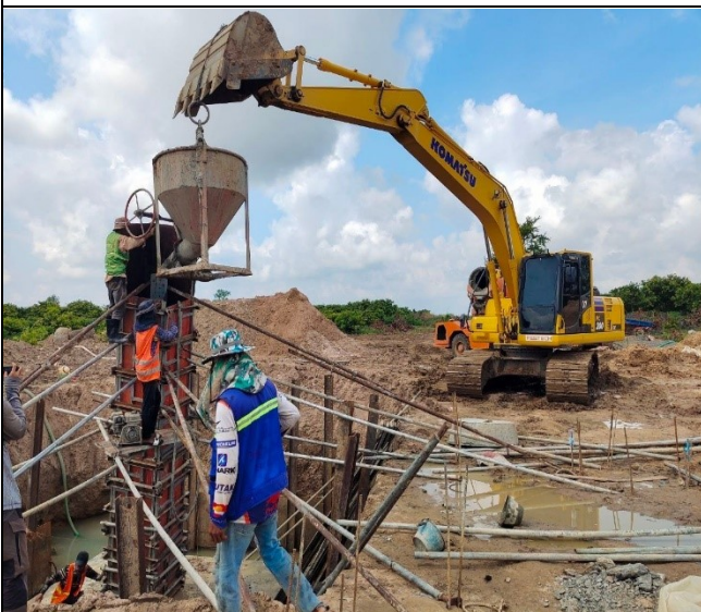
Chimney concrete leg D
