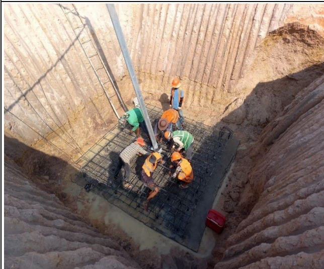
Base rebar installation leg B
