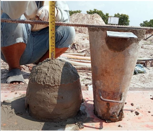
Chimney concrete leg B
