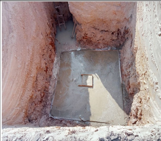
Lean concrete leg B
