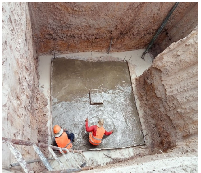
Lean concrete leg C
