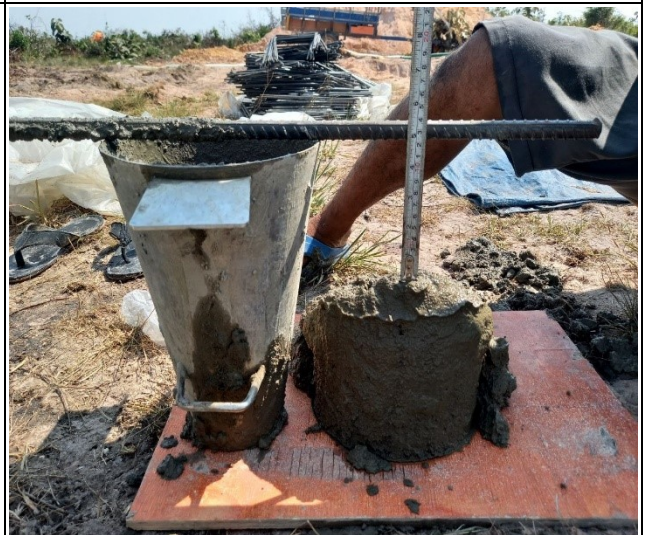
Slump teste for casting base leg B
