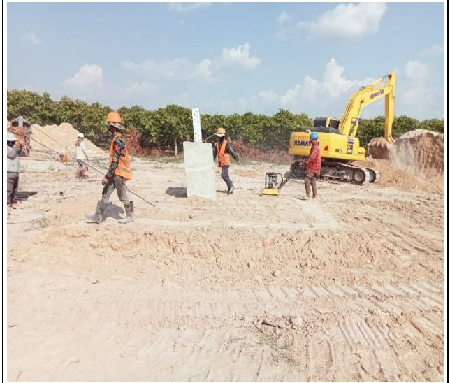
Backfill leg A, D
