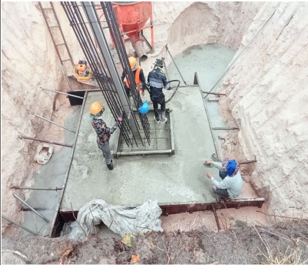
Base concrete leg B
