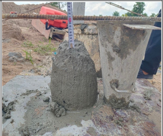
Slump testing leg D
