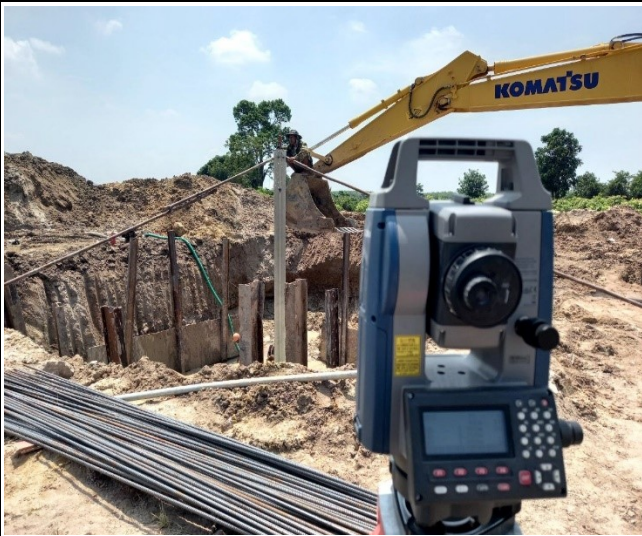
Stub setting leg C
