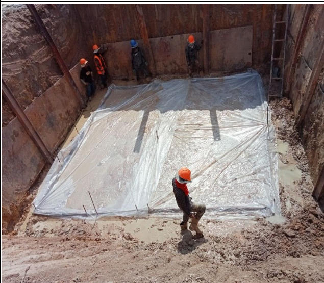
Lean concrete leg D
