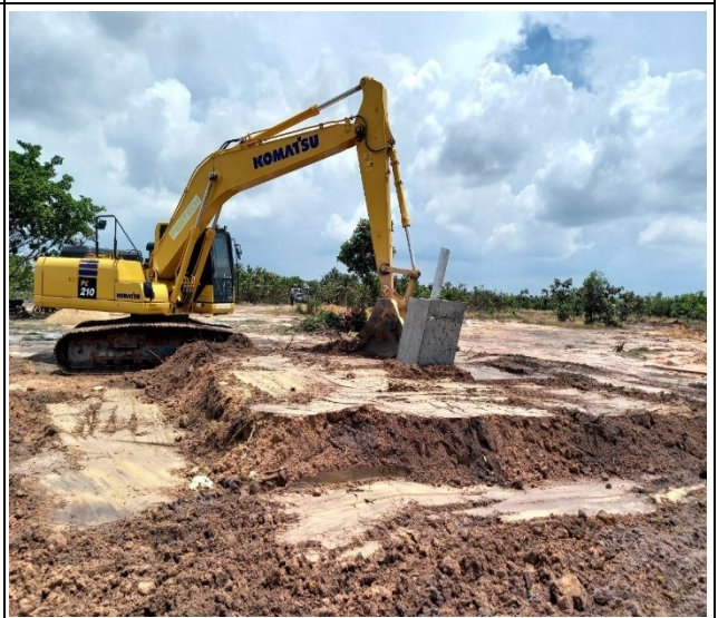
Backfill leg A
