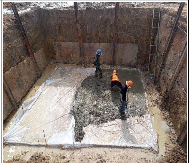
Lean concrete leg D
