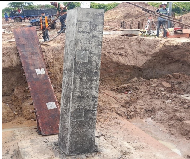
Remove form box leg C
