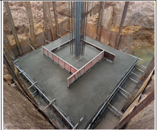
Base concrete leg A
