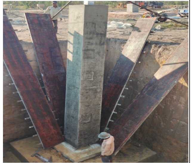
Remove chimney form box leg D
