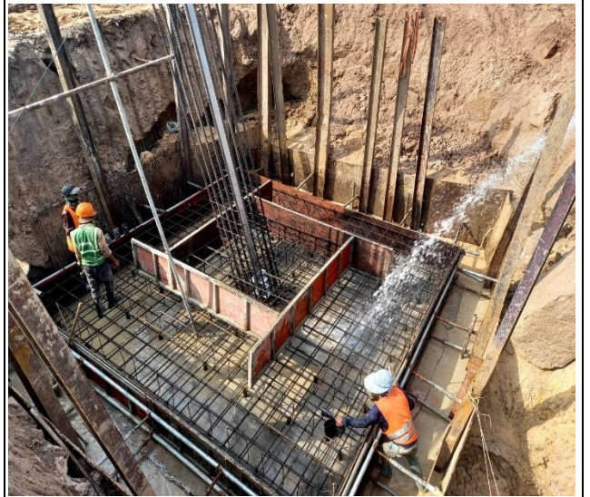
Base concrete leg A
