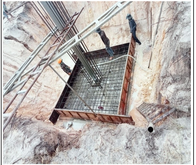
Base rebar & formwork installation leg A
