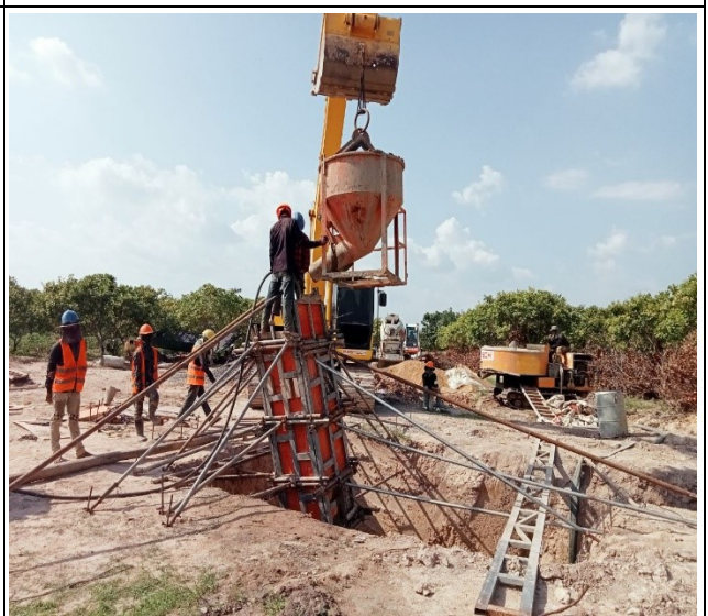
Chimney concrete leg D
