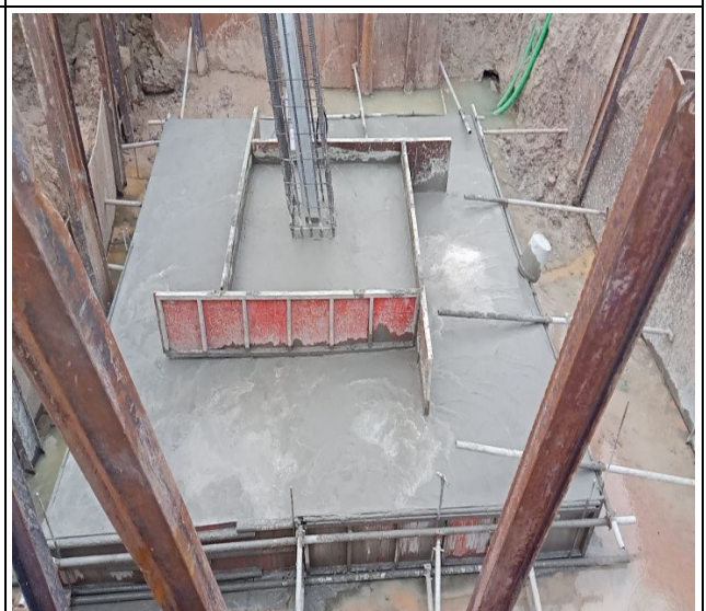
Base concrete leg C
