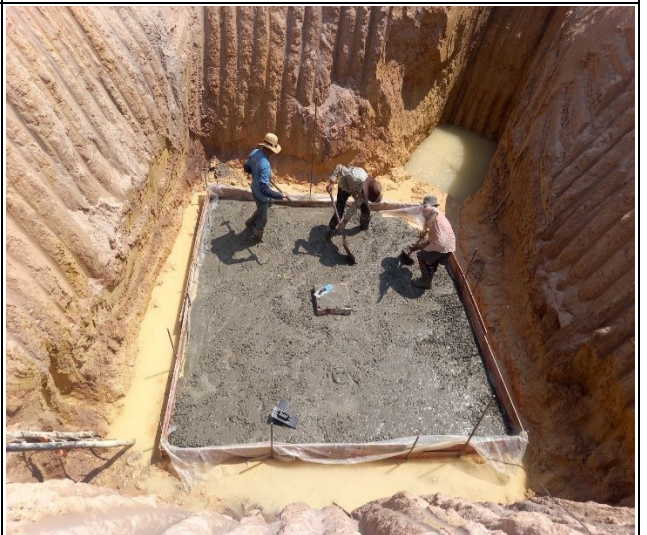
Lean concrete leg A
