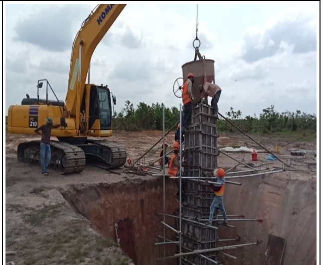
Chimney concrete leg A
