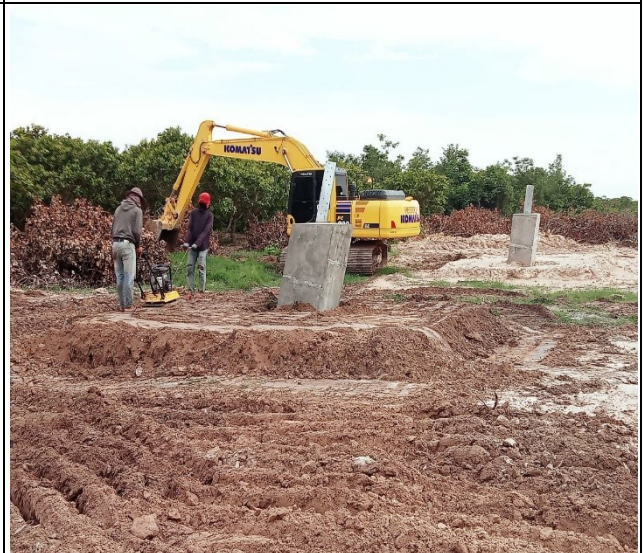
Backfill leg C
