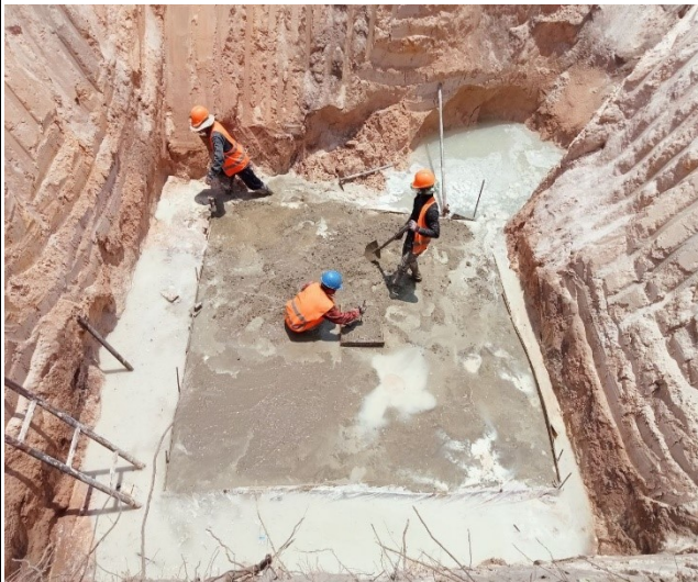
Lean concrete leg B
