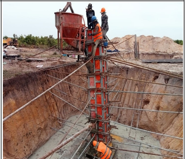
Chimney concrete leg C
