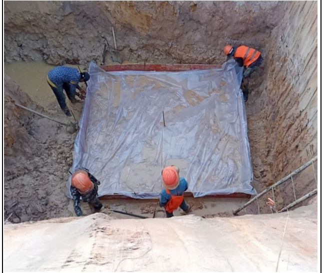
Lean concrete leg A
