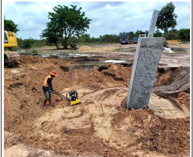
Backfill leg A
