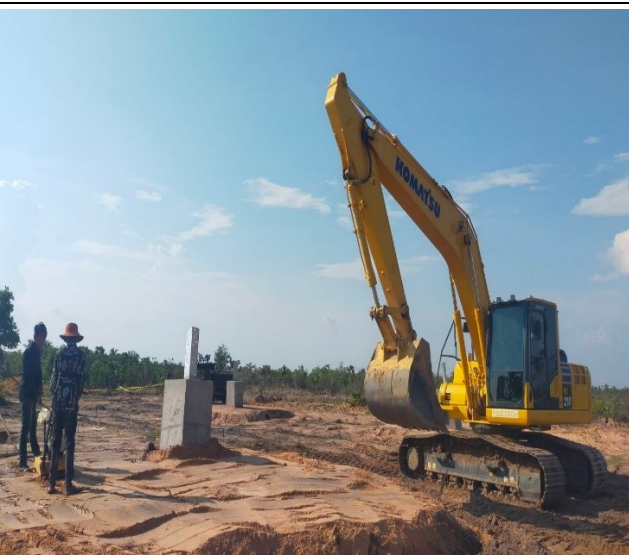
Backfill leg D
