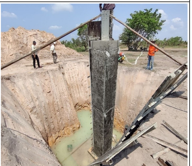
Remove chimney form box leg A
