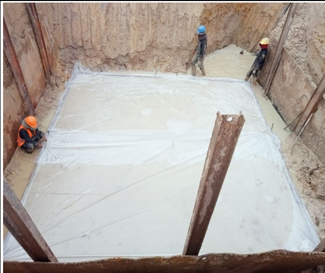
Lean concrete leg A
