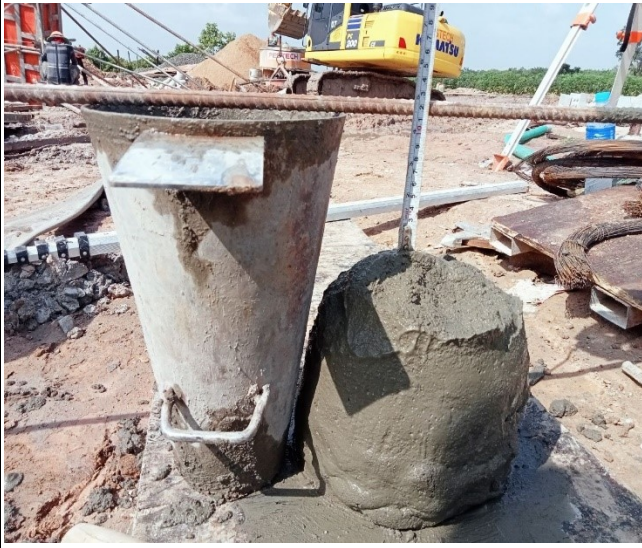
Slump testing leg D
