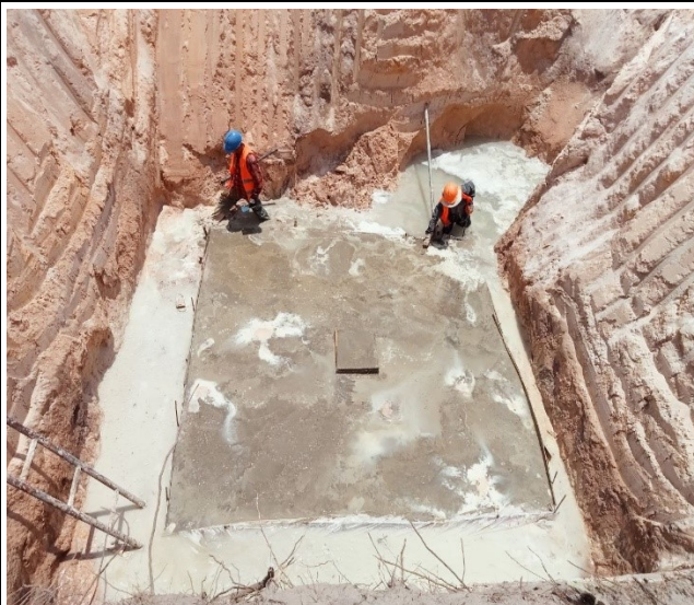
Lean concrete leg B
