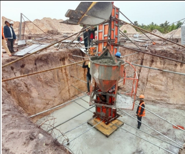
Chimney concrete leg D
