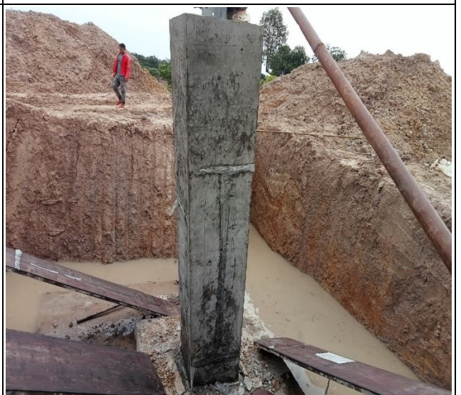
Chimney concrete leg D
