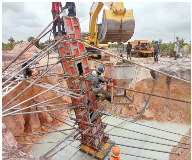
Chimney concrete leg A
