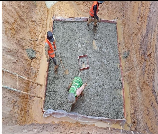
Lean concrete leg D
