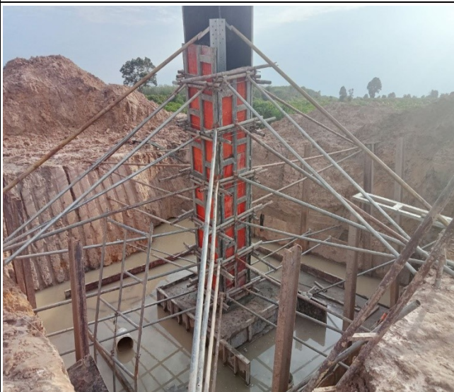
Chimney concrete leg A
