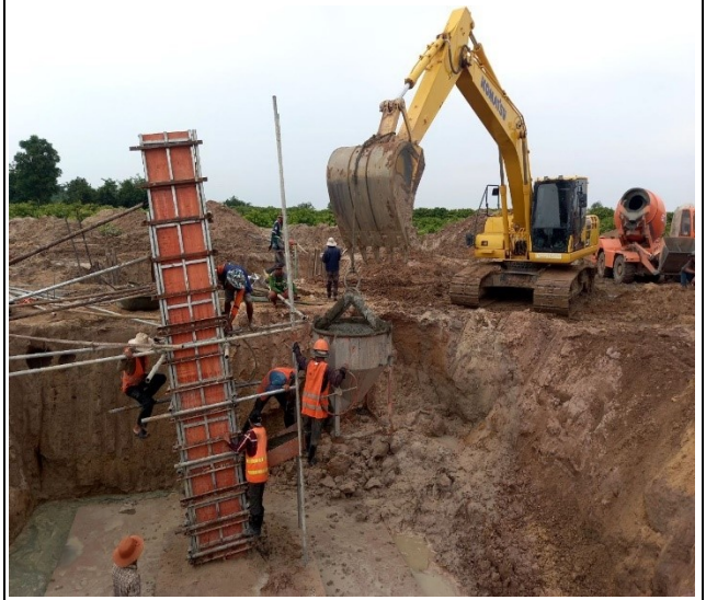
Chimney concrete leg A
