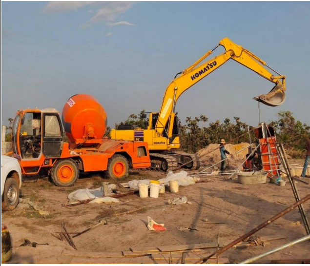
Chimney concrete leg D
