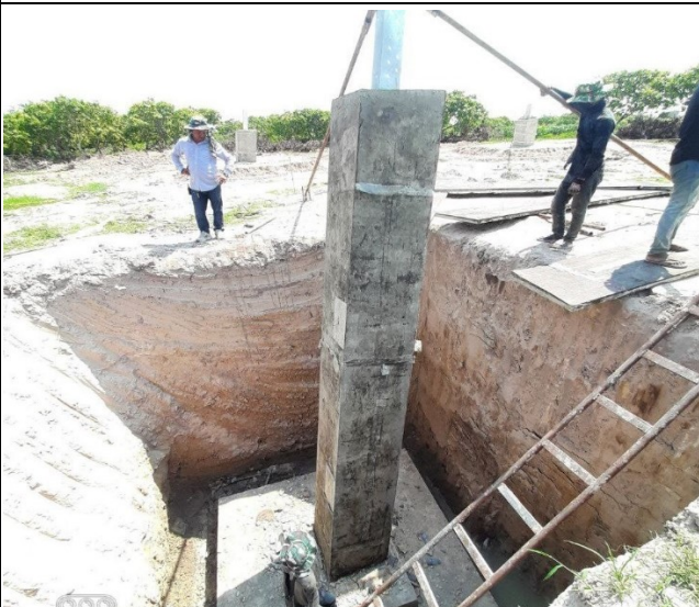
Remove chimney form box leg C
