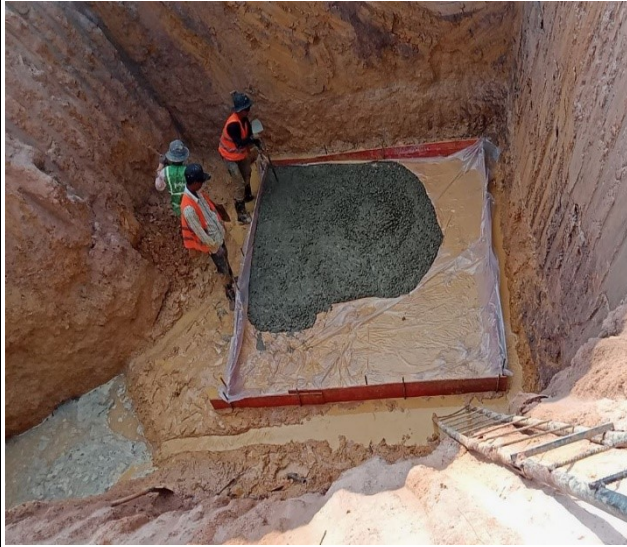
Lean concrete leg D
