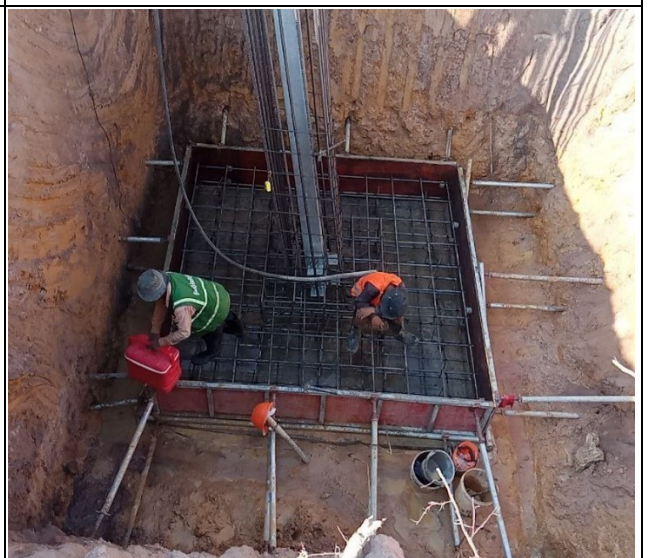
Base rebar & formwork installation leg D.
