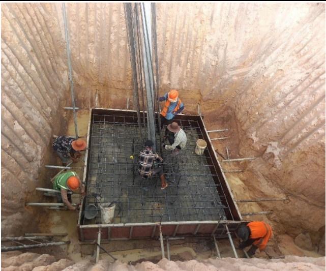
Base rebar installation leg A
