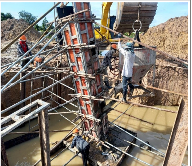
Chimney concrete leg A
