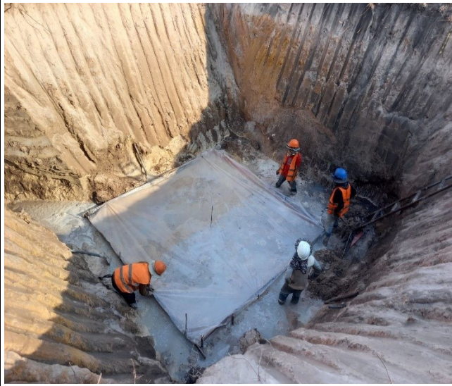
Lean concrete leg C
