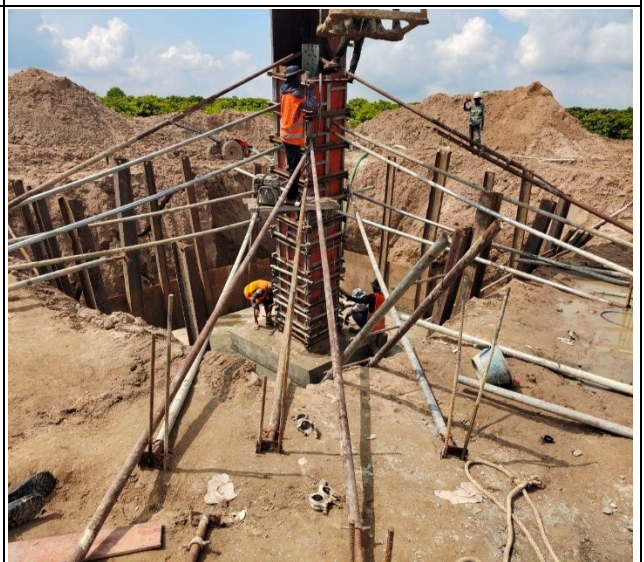
Chimney concrete leg D
