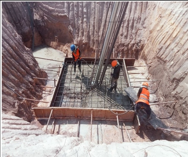
Base concrete leg C
