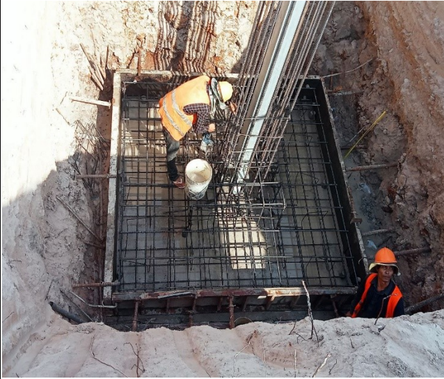
Base concrete leg B
