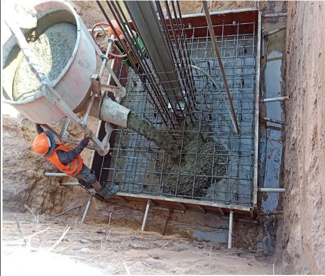
Base concrete leg D.
