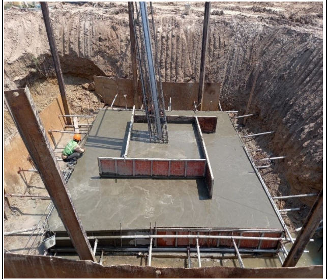
Base concrete leg B
