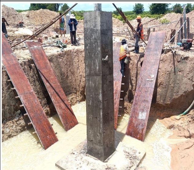
Chimney concrete leg A
