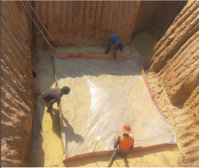
Lean concrete leg B
