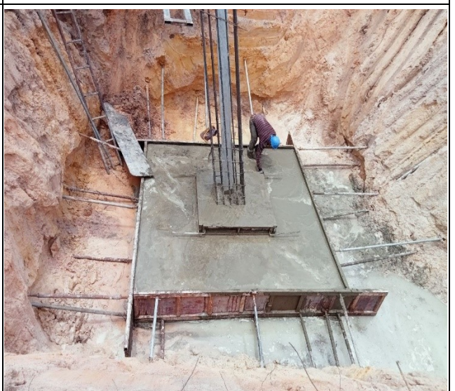
Base concrete leg A
