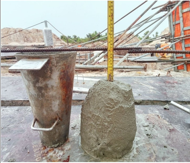
Slump testing leg D
