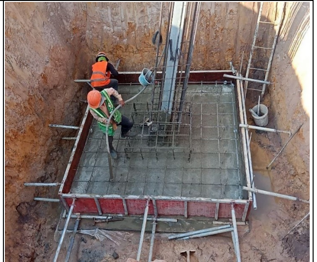
Base concrete leg A.
