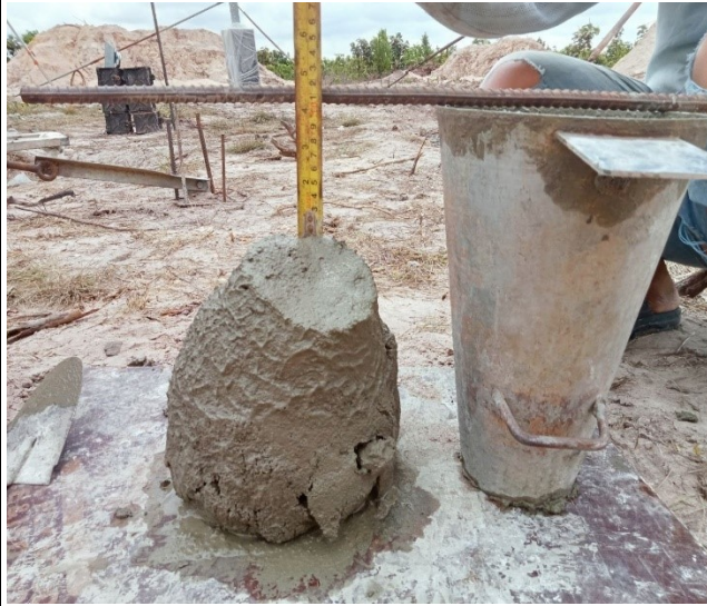
Slump testing leg A
