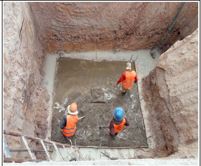
Lean concrete leg C
