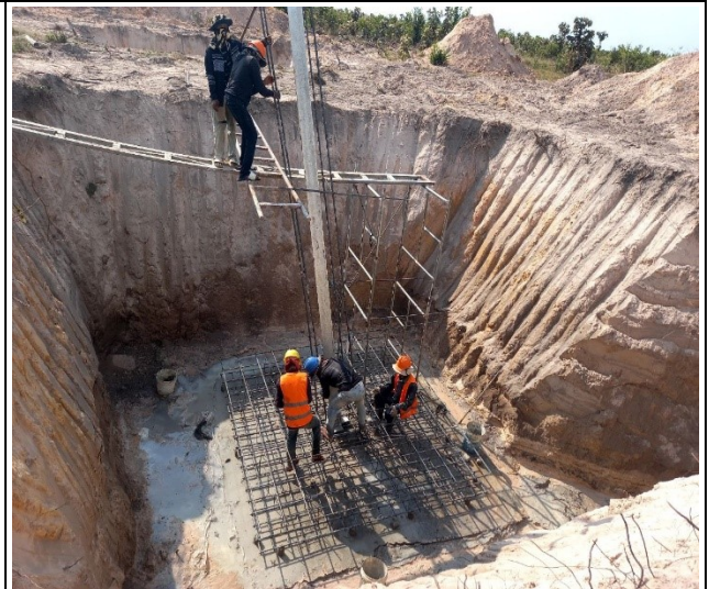
Base rebar & formwork installation leg C
