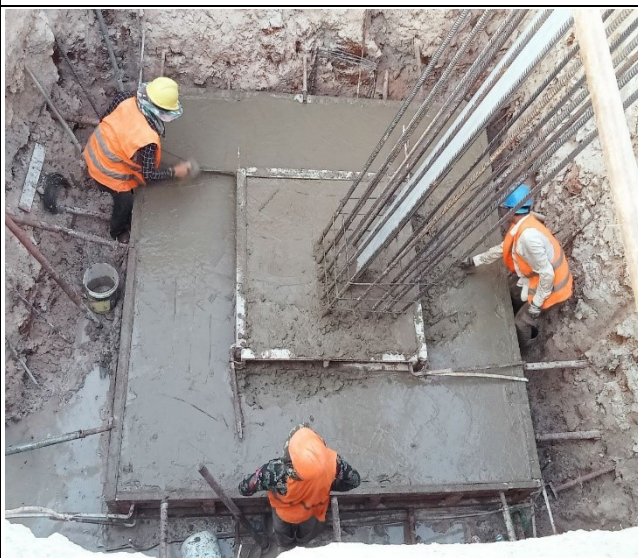
Base concrete leg B
