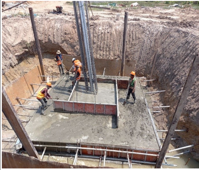
Base concrete leg B
