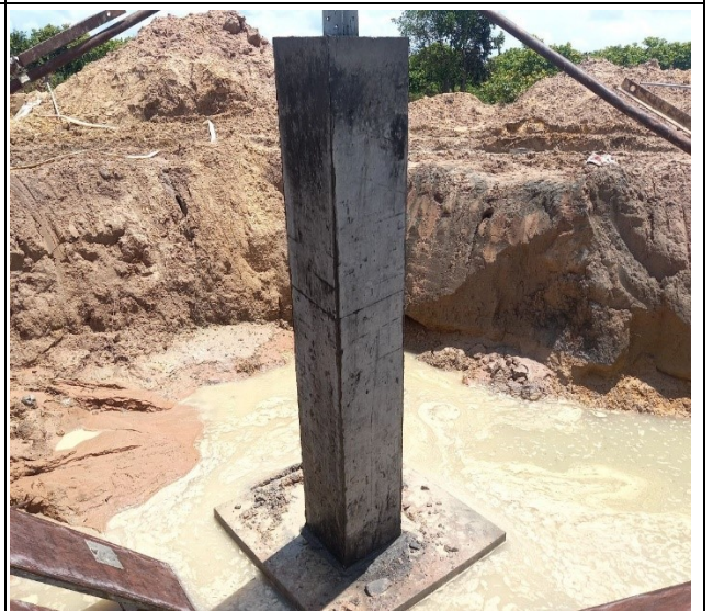
Chimney concrete leg A
