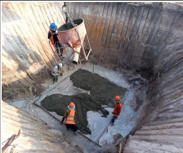
Lean concrete leg C
