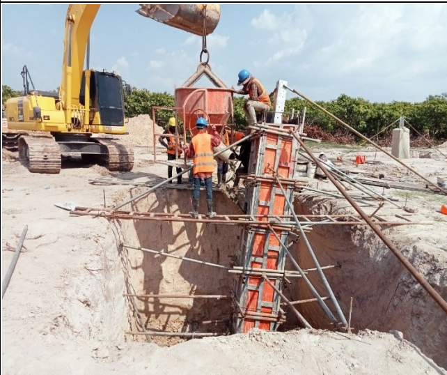
Chimney concrete leg B
