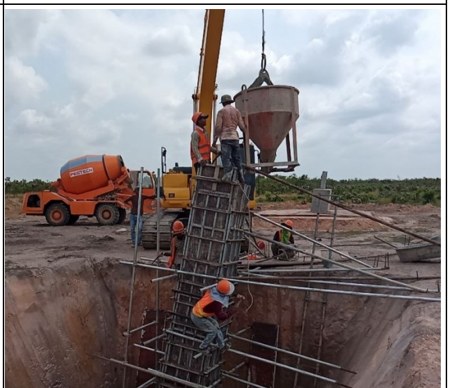
Chimney concrete leg A
