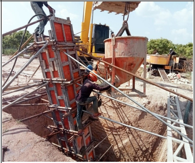
Chimney concrete leg D
