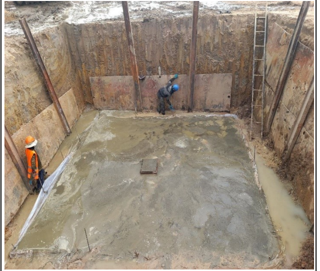
Lean concrete leg D
