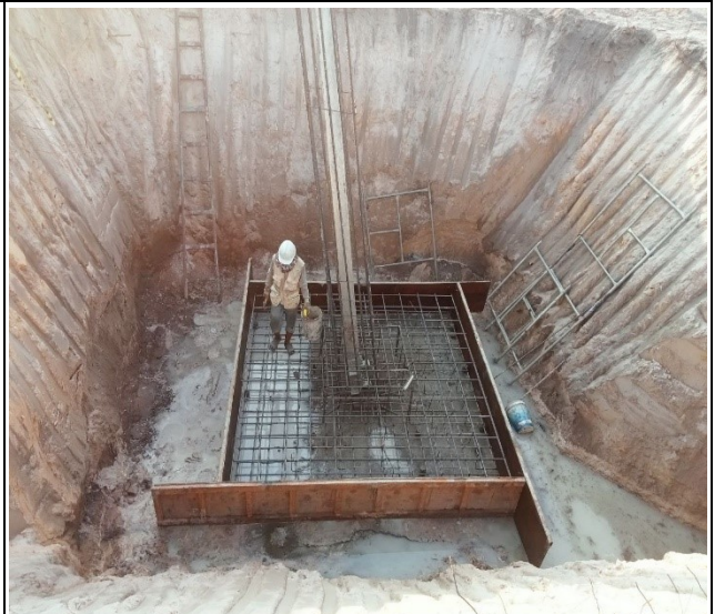
formwork installation leg C
