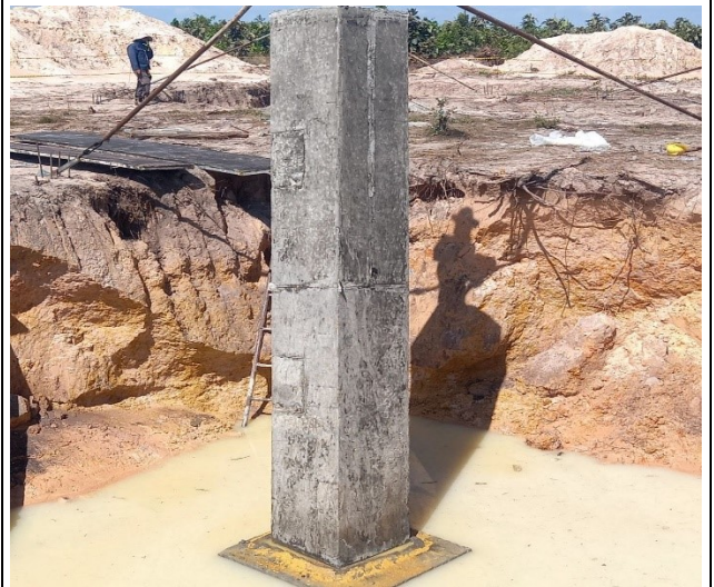
Remove chimney form box leg A
