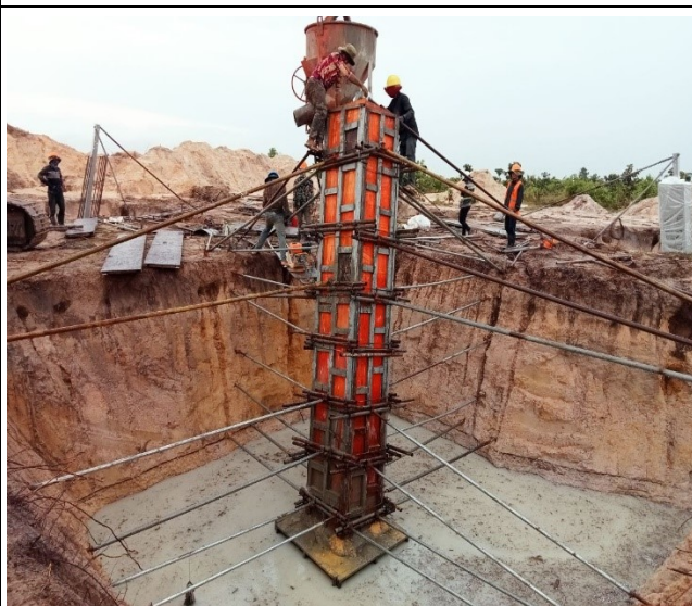
Chimney concrete leg D
