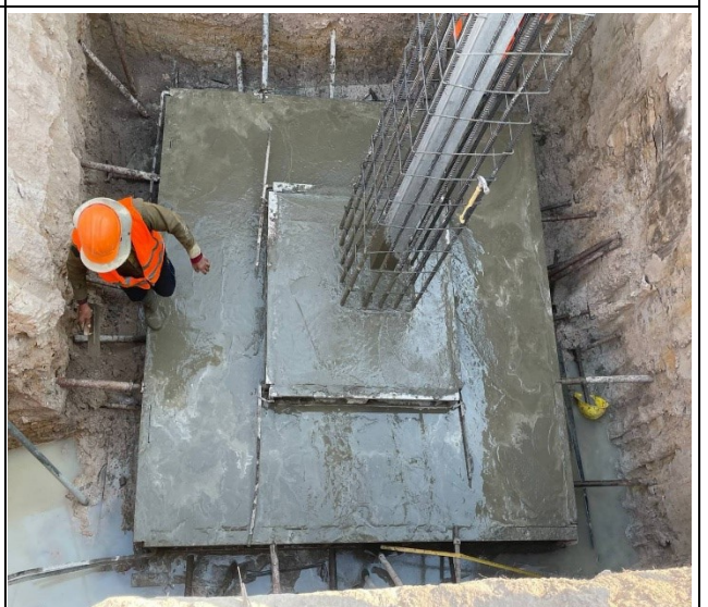
Base concrete leg C
