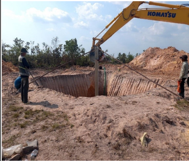
Lean concrete leg B
