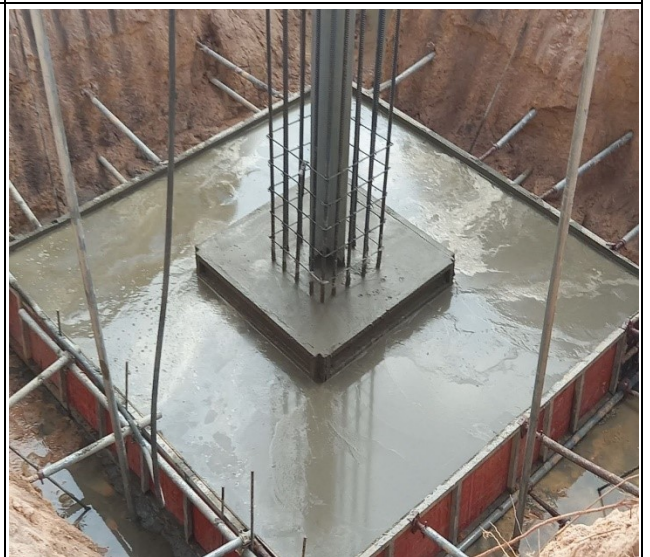
Base casting concrete leg B
