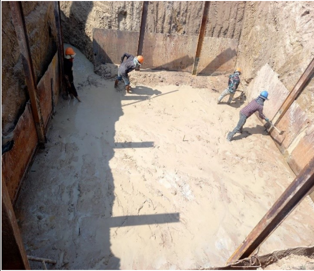
Lean concrete leg C
