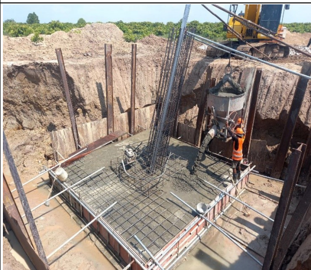
Base concrete leg C
