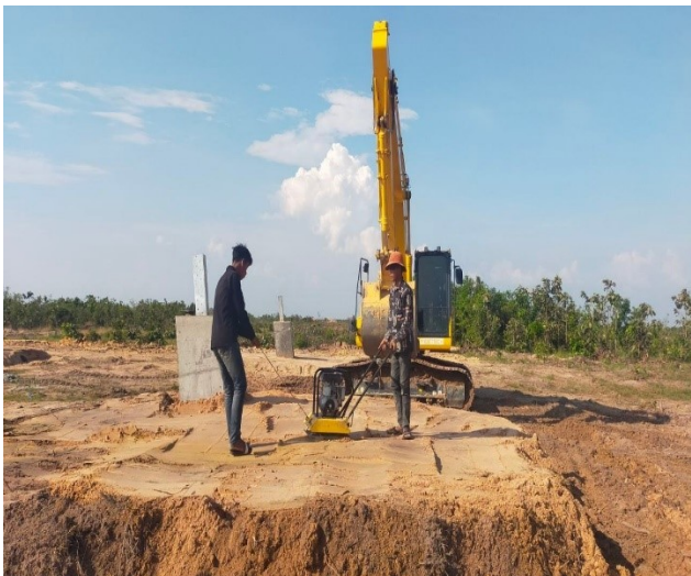
Backfill leg D
