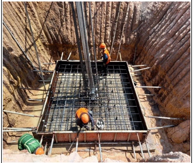
Base formwork installation leg B
