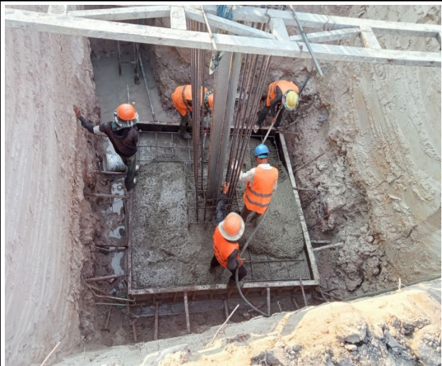
Base concrete leg B
