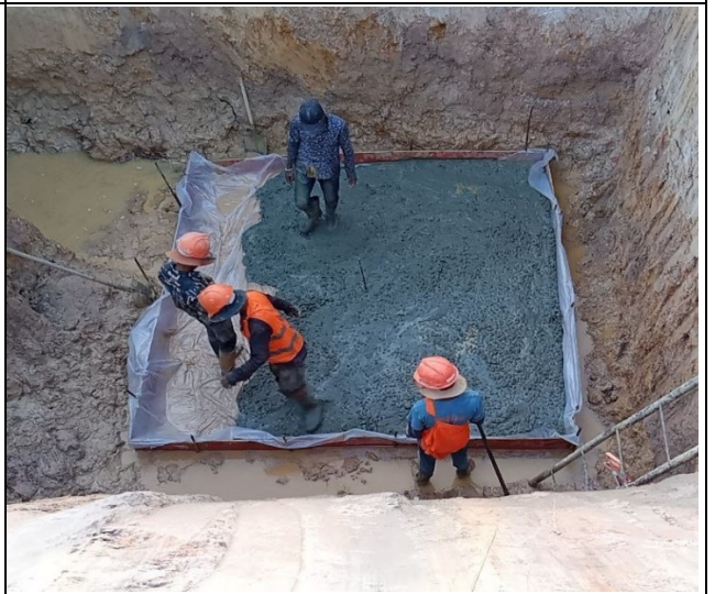
Lean concrete leg A
