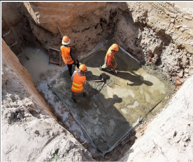
Lean concrete leg B
