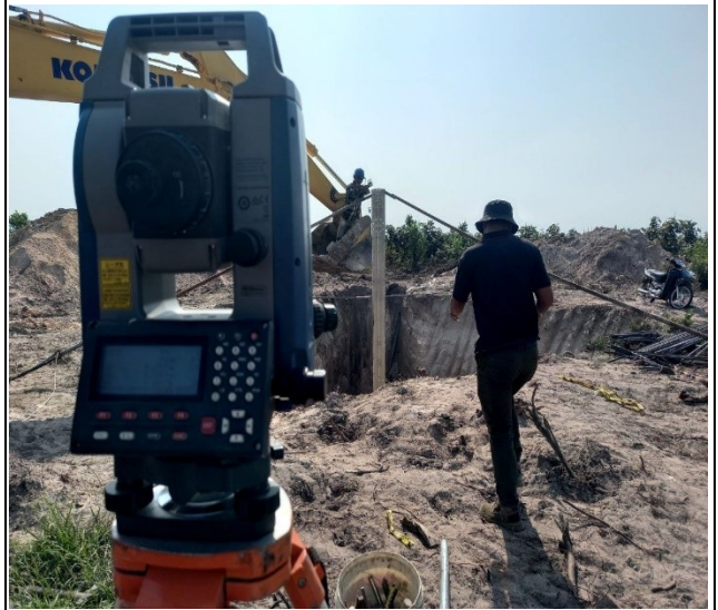
Stub setting leg C
