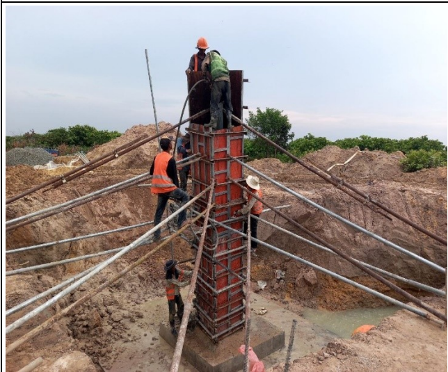
Chimney concrete leg A
