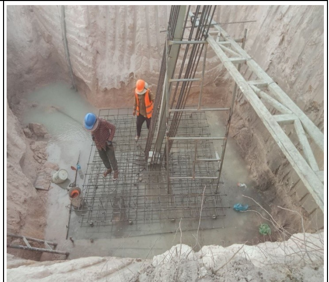
Base rebar installation leg B
