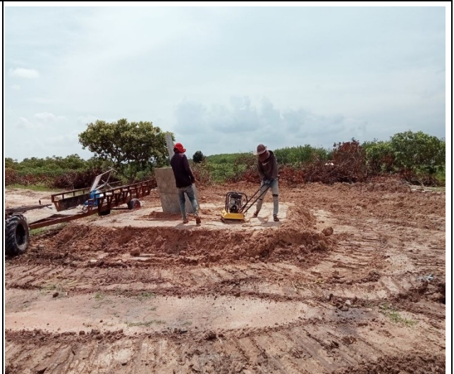
Backfill leg A
