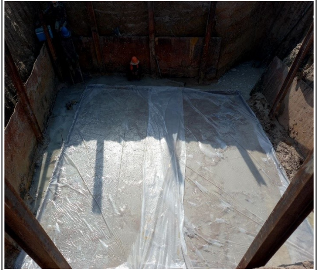
Lean concrete leg C
