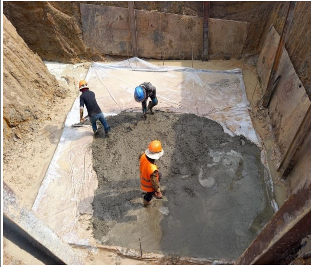
Lean concrete leg D
