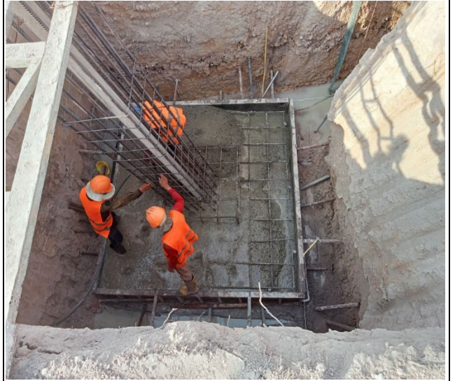
Base concrete leg C
