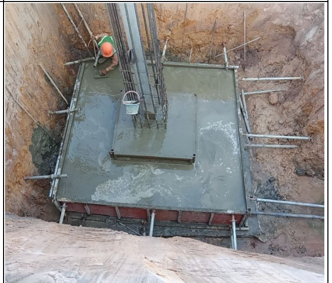
Base concrete leg A.
