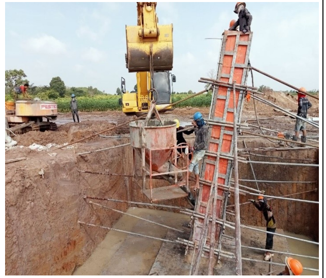
Chimney concrete leg D
