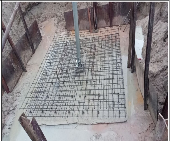
Rebar installation leg C
