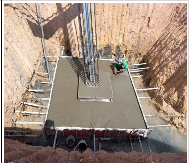
Base casting concrete leg A
