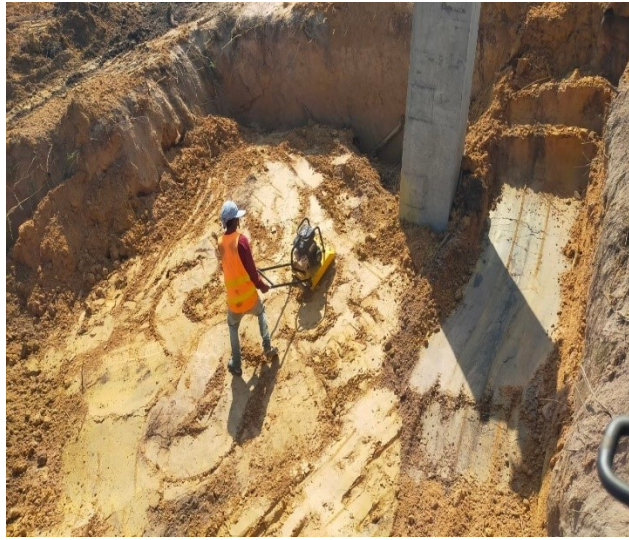
Backfill leg D
