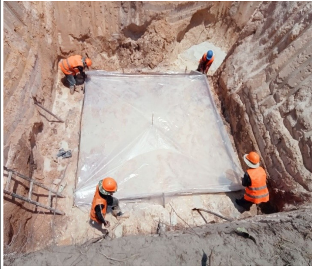
Lean concrete leg B
