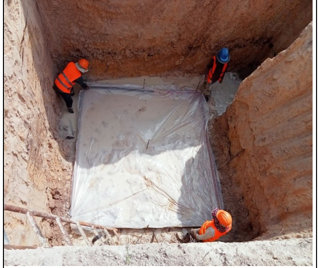
Lean concrete leg C
