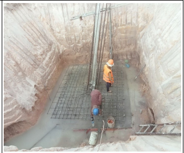
Base rebar installation leg B
