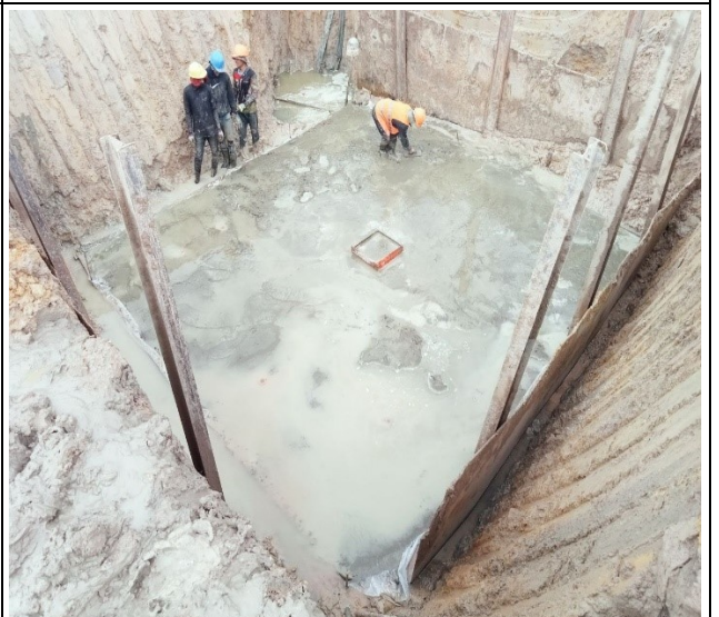
Lean concrete leg A
