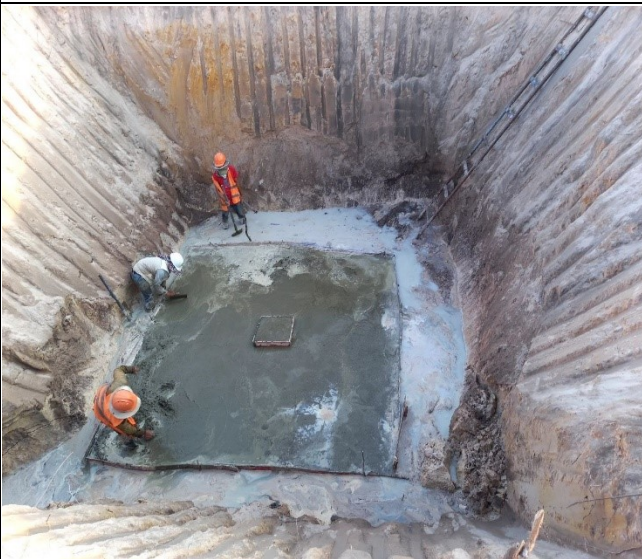
Lean concrete leg C
