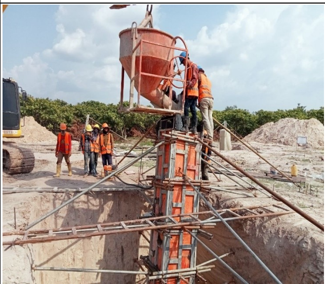
Chimney concrete leg B
