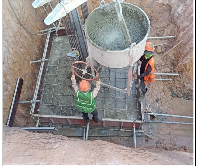
Base concrete leg A.
