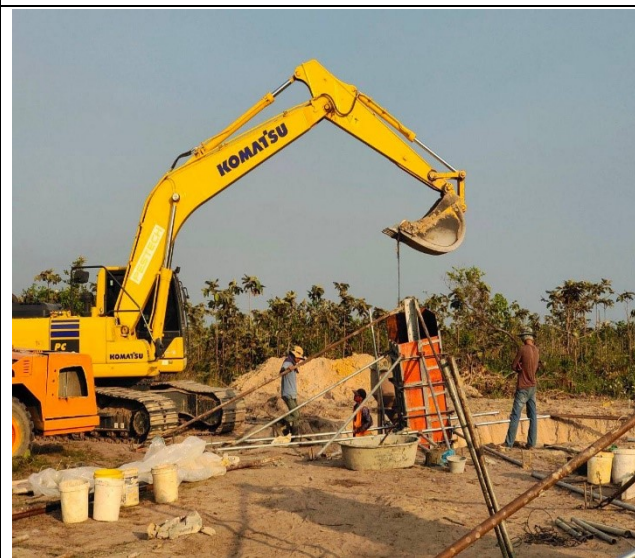
Chimney concrete leg D
