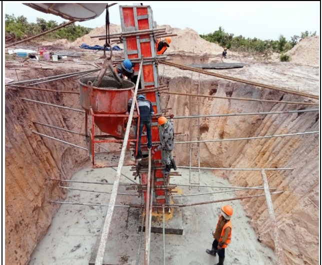
Chimney concrete leg C
