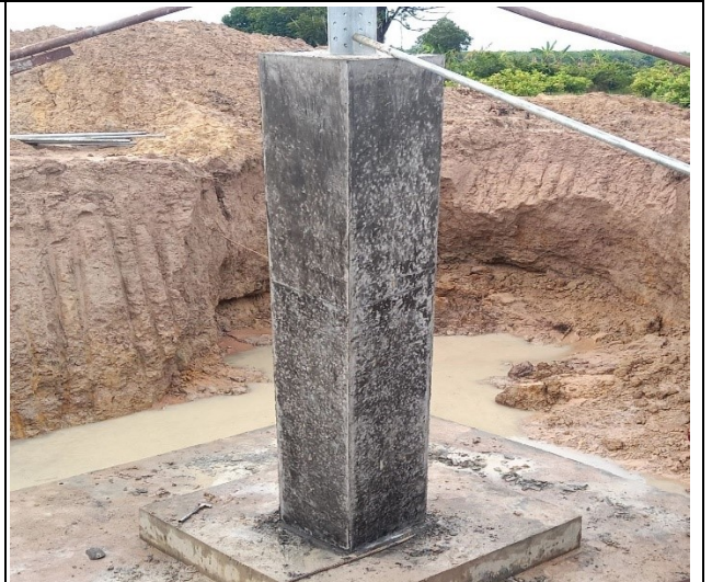
Remove form box leg C
