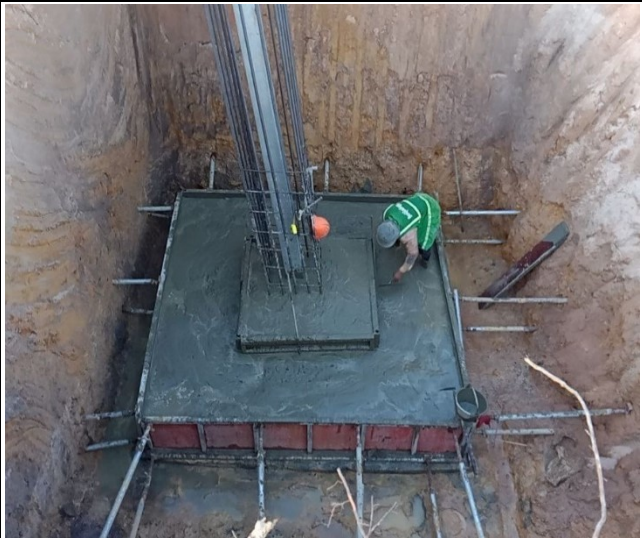
Base concrete leg D.
