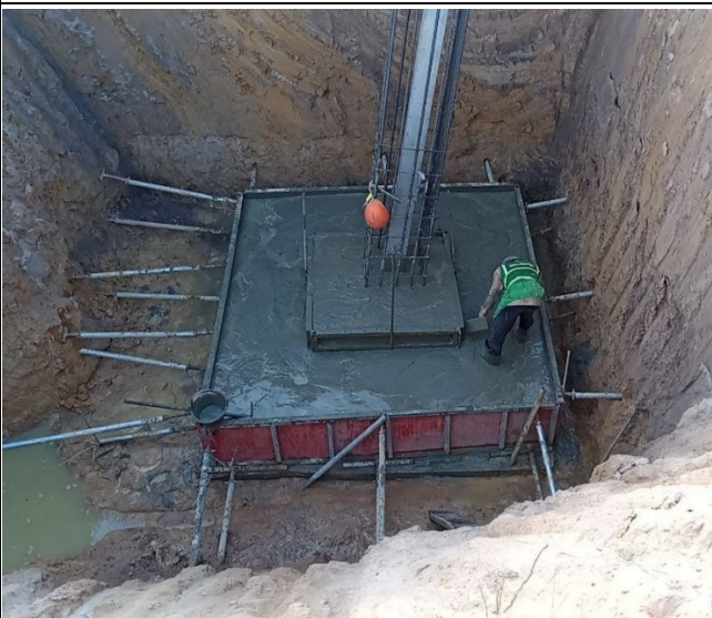
Base concrete leg D.
