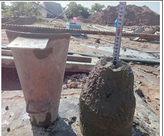
Slump testing leg A
