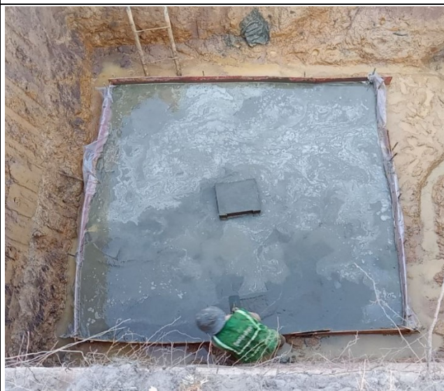
Lean concrete leg D
