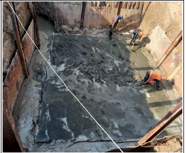
Lean concrete leg C
