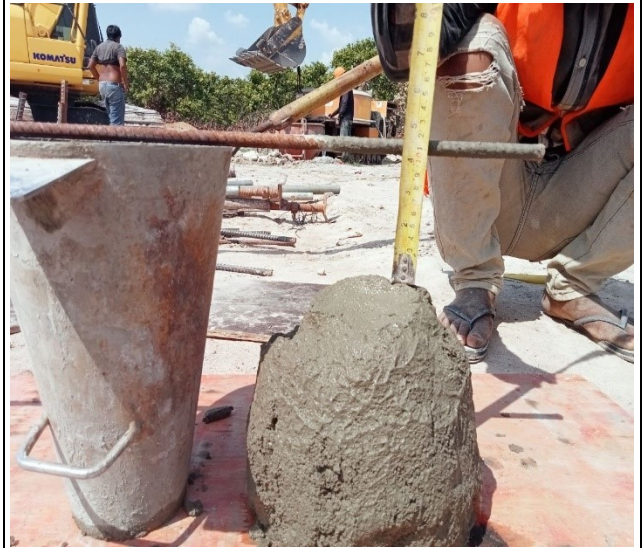
Chimney concrete leg D
