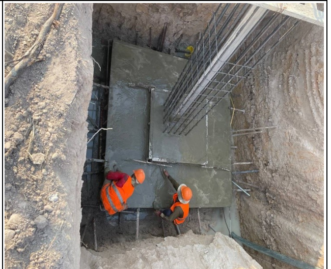
Base concrete leg C
