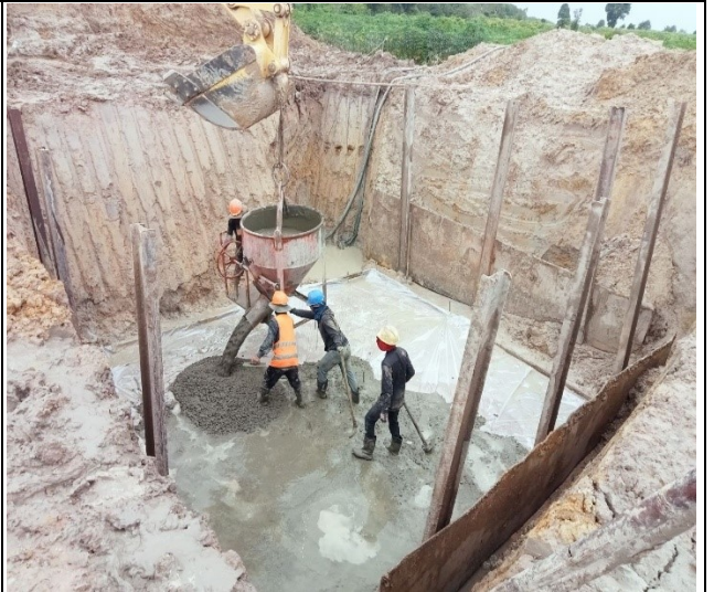
Lean concrete leg A
