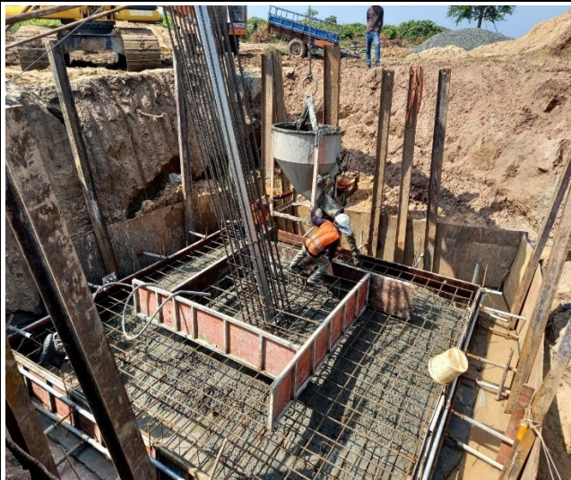
Base concrete leg A
