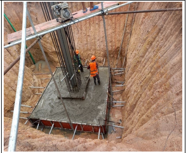
Base casting concrete leg A
