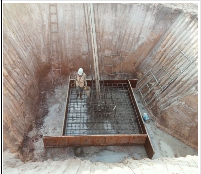
Base rebar & formwork installation leg C
