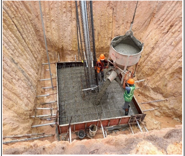
Base casting concrete leg A
