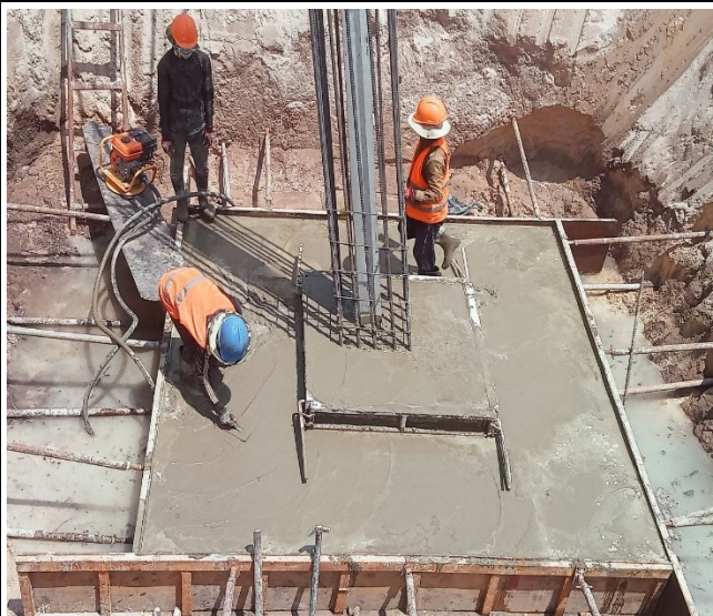
Base concrete leg C
