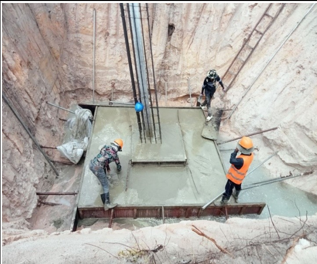
Base concrete leg B
