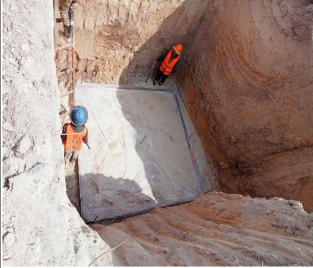
Lean concrete leg B
