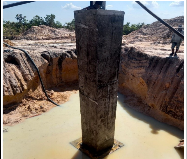
Remove chimney form box leg A
