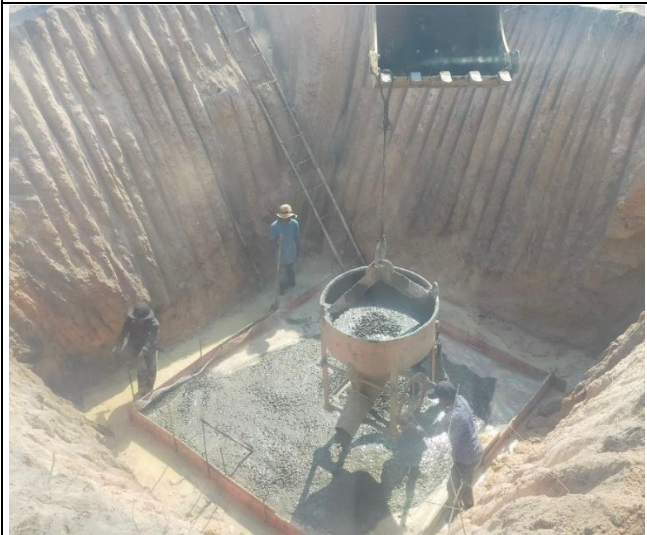
Lean concrete leg B
