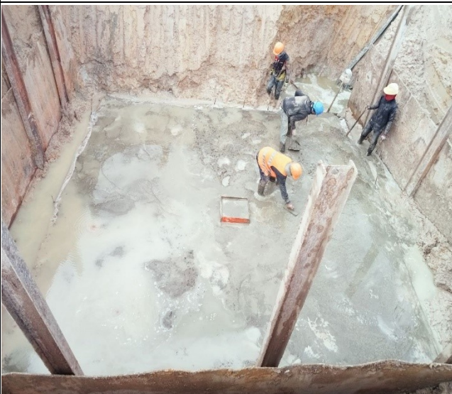
Lean concrete leg A
