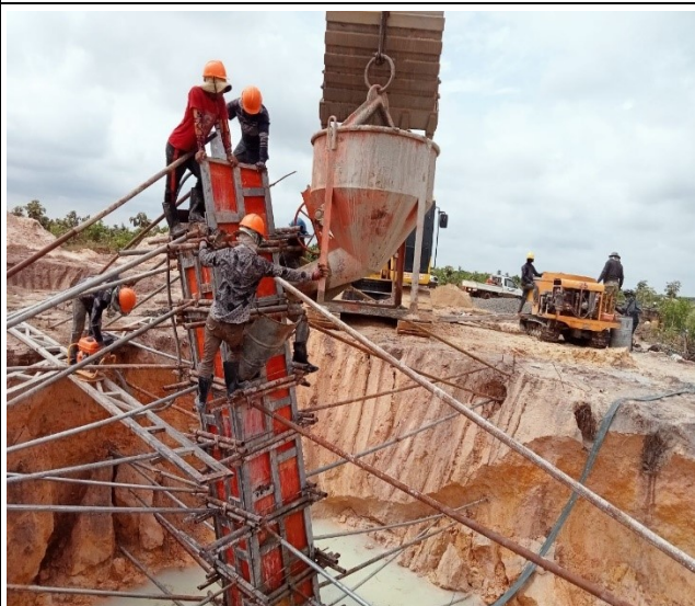
Chimney concrete leg A
