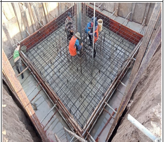
Base concrete leg D
