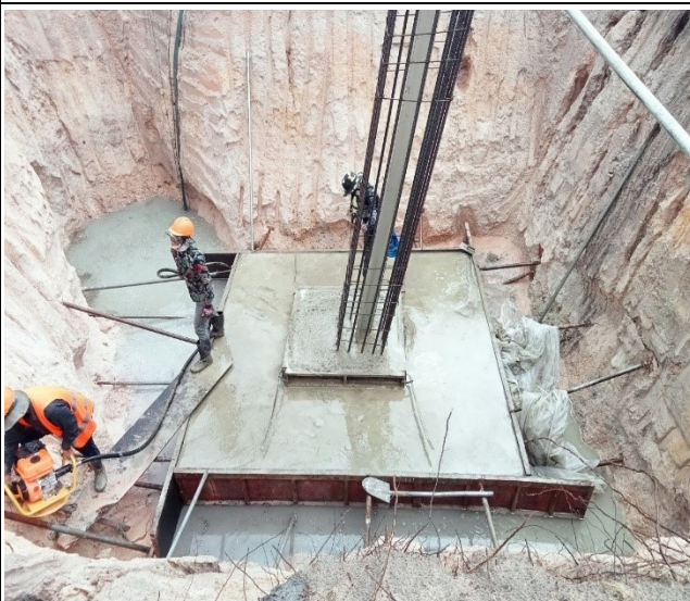
Base concrete leg B
