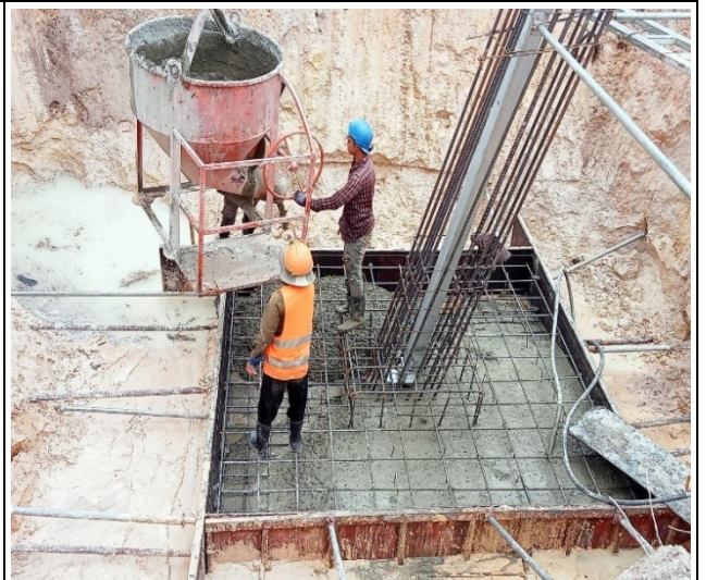
Base concrete leg A
