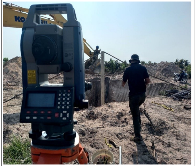
Stub setting leg C
