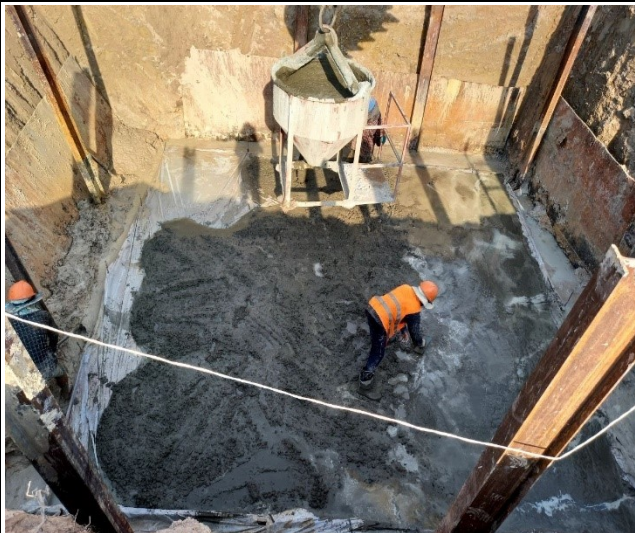
Lean concrete leg C
